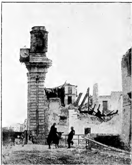
FIG. 110.—Messina-Reggio earthquake of December 28, 1908. A wrecked house on Via Porta Imperiale, Messina. The clock on the corner post indicates the time of occurrence of the earthquake, 5.20 a.m. (From the Bulletin of the Imperial Earthquake Investigation Committee, Tokyo, November, 1909. )
