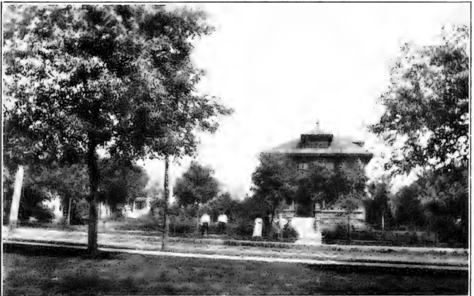
Residence of Fred Stalley, Moorhead
