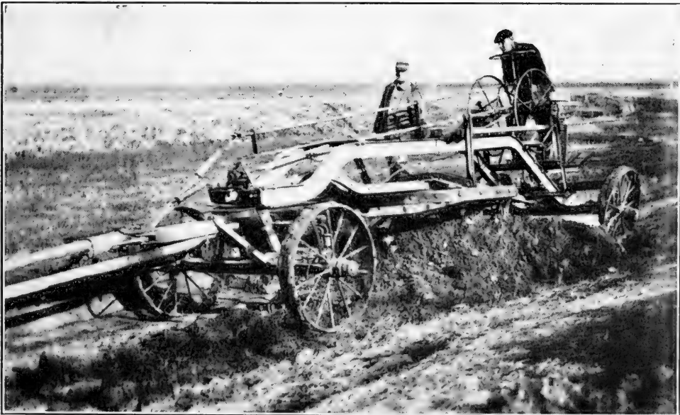
Push Grader Throwing Up Grade on State Road
