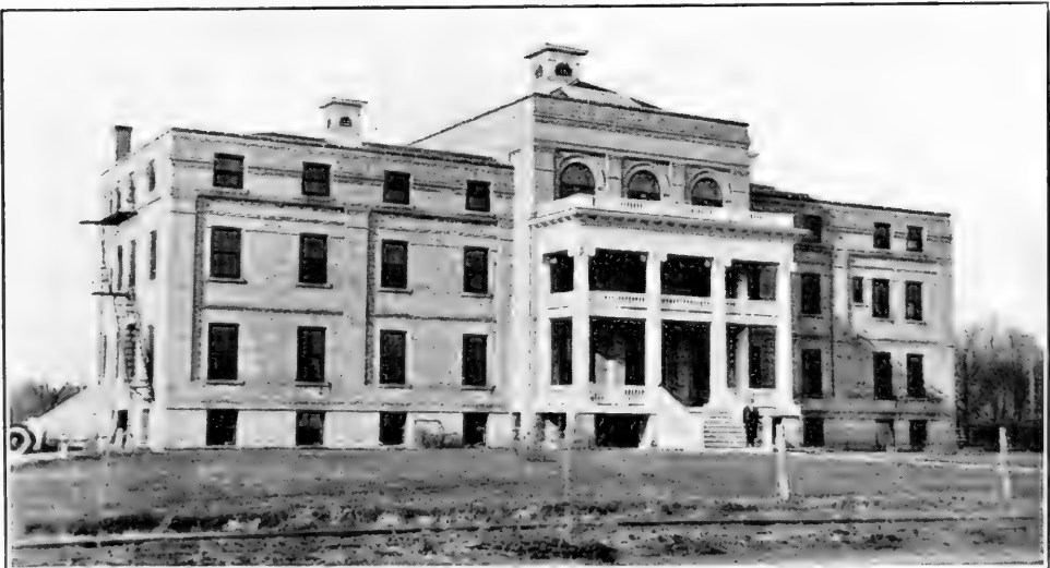
Northwestern Hospital, Moorhead
