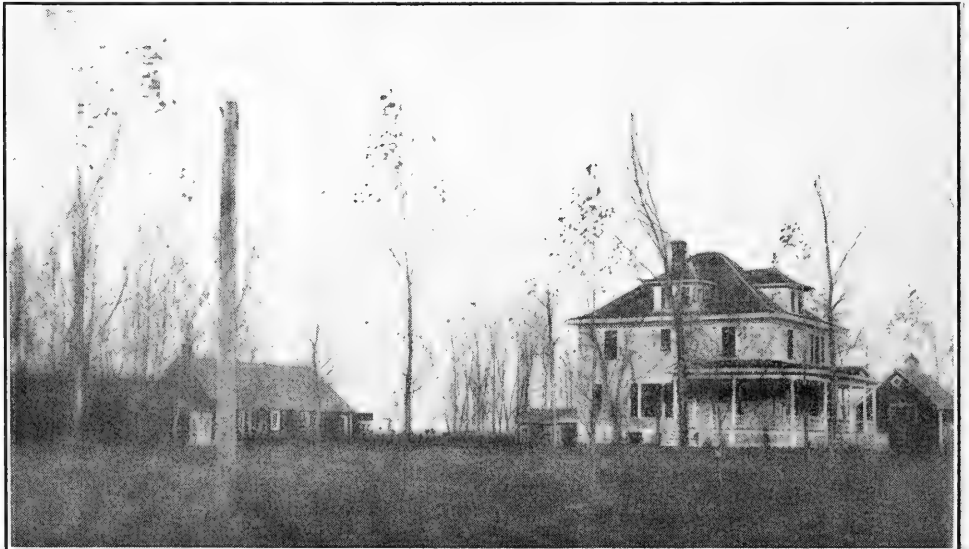
Modern Buildings on Fred H. Kuehl Farm, Glyndon Township
