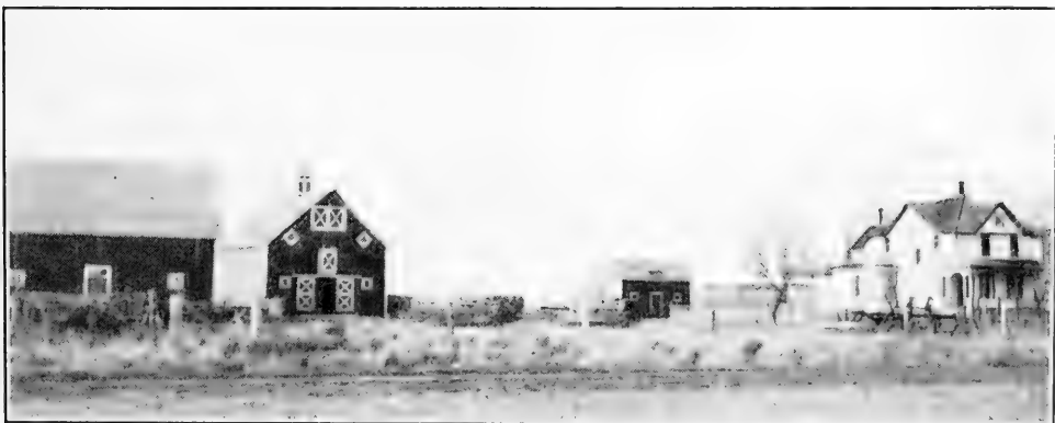
Part of Frank P. Thompson Farmstead, Alliance Township
