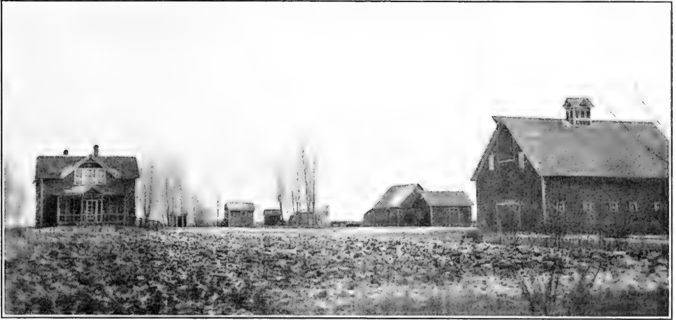
Residence and Buildings on August Hoppe Farm, Alliance Township
