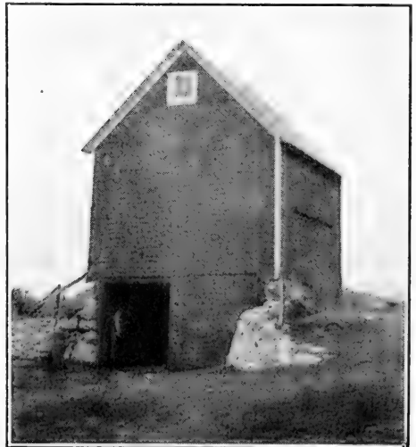
Elevator on T. T. Woodward Farm
