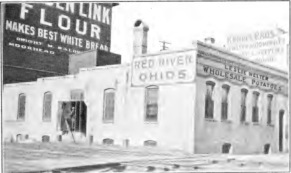
Leslie Welter's Potato Cellar and Warehouse, Moorhead
