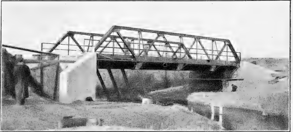
Bridge on State Road Near Manitoba Junction
