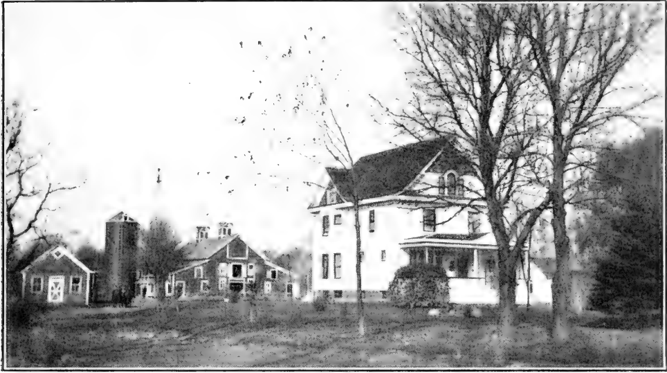
Coming Up the Driveway on the Otto J. Grover Farm
