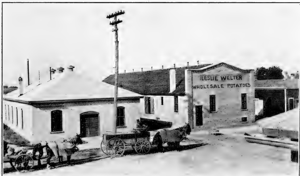
Leslie Welter's Potato House—Ventilators from Cellar Through Roof
