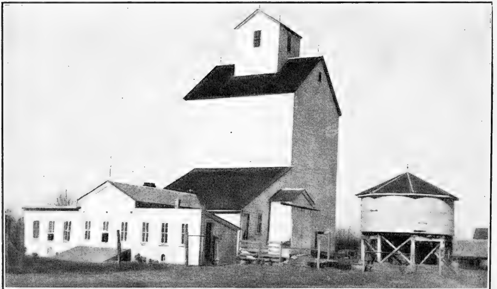
Elevator Where Grain Is Stored, Cleaned and Ground on the E. D. Grant Farm
