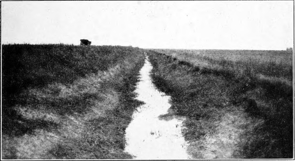
One of the Clay County Drainage Ditches—Automobile on Grade at Left
