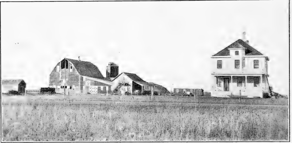
The Frank Kimm Farmstead in Oakport Township
