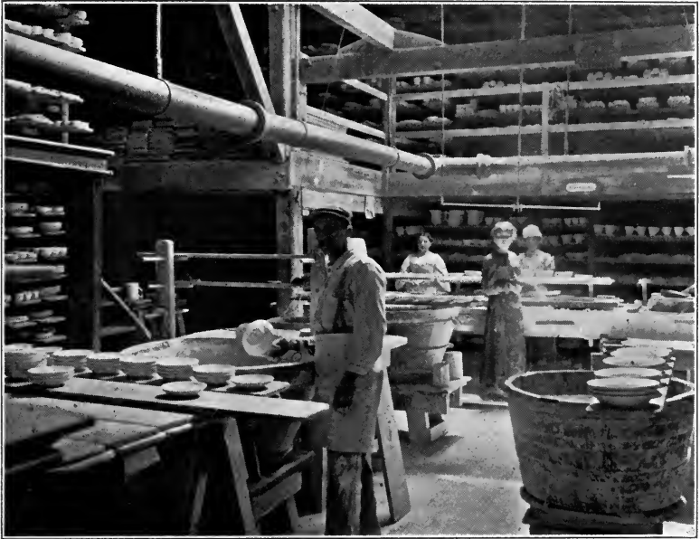
Dipping bisuit ware into the glazing-tubs. (Photo by H. Ries.)
