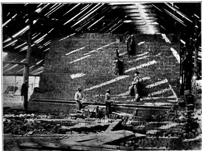
FIG. 2.—Setting brick for a scove-kiln. (After H. Ries, N. J. Geol. Surv., Fin. Rept., VI, p. 240, 1900. )
