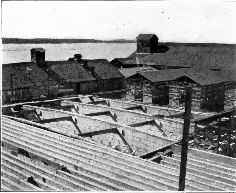
FIG. 1.—View showing portion of sand-troughs, settling-tanks, and drying-racks at a kaolin-washing plant. (After Ries, Md. Geol. Surv., IV, p. 270, 1902.)
