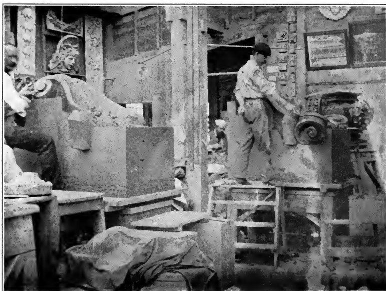
FIG. 2.—Modeling terra-cotta objects. (Photo by H. Ries.)
