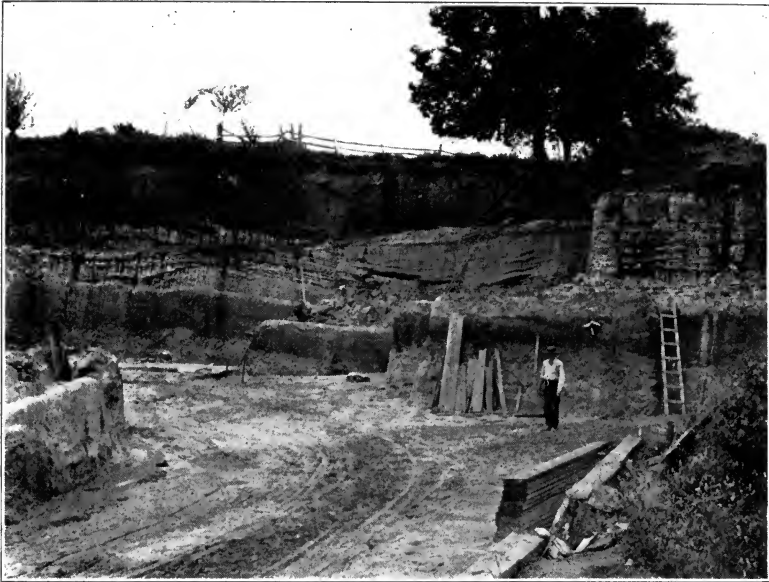
FIG. 1.—Section showing beds of stratified clay overlain by glacial drift. (After Ries, N. J. Geol. Surv., Fin. Rept., VI, p. 440.)
