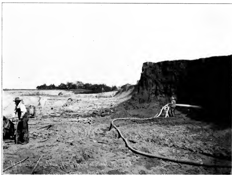
FIG. 2.—Removing the overburden from a shale-bed by hydraulicking. Photo loaned by Illinois Geological Survey.)
