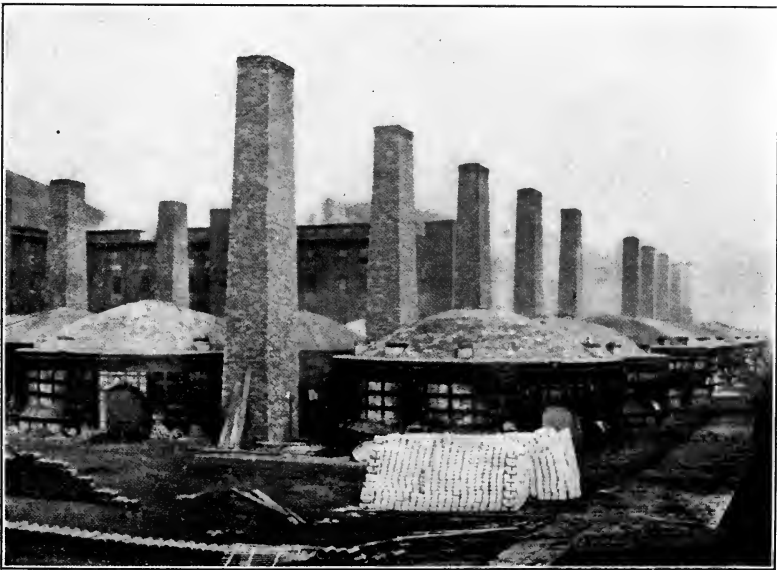
FIG. 2.—Down-draft kilns. (Photo loaned by Robinson Clay-product Co.)
