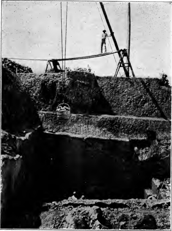
Showing method of working clay in a rectangular pit. (After Ries, N. J. Geol. Surv., Fin. Rept., VI, p. 34, 1904. )
