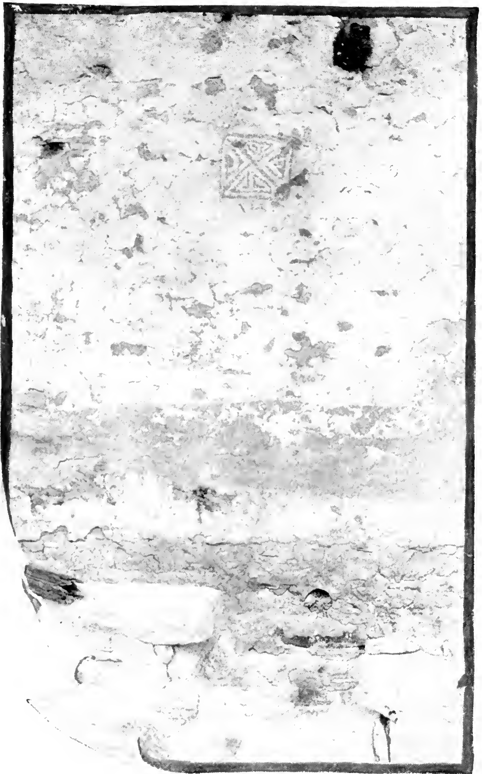
PLASTERED AND PAINTED WALL.
