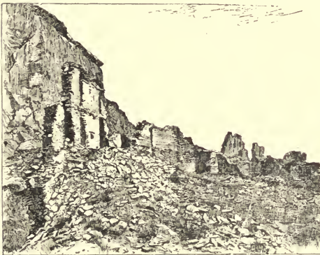
RUINED HOUSE IN CHACO CANYON.
