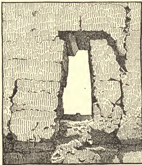
FIG. 5. NORTH WALL OF NORTH ROOM
