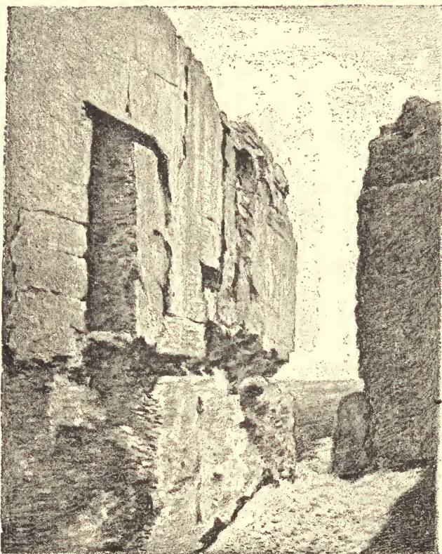
FIG. 4. EAST WALL OF NORTH ROOM
