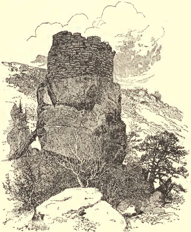
FIG. 2. BLACK TOWER ON THE MANCOS
