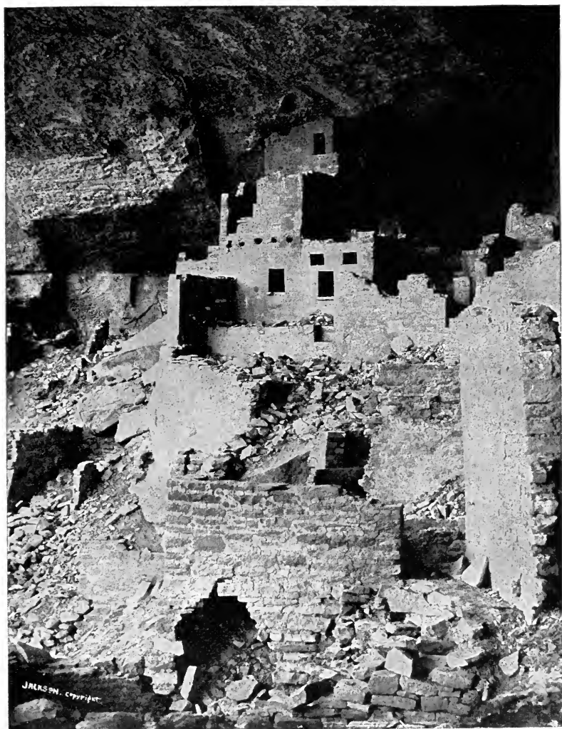
VIEW SHOWING TERRACES AND DIFFERENT STORIES.
