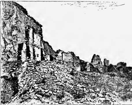
RUINED HOUSE IN CHACO CANYON.
