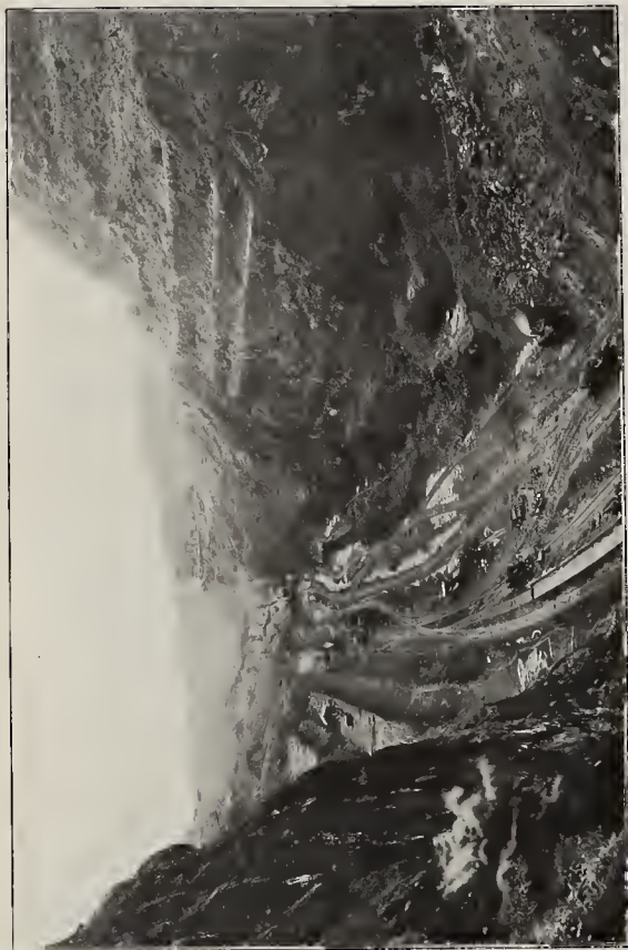
GAILLARD CUT. DEEPEST EXCAVATED PORTION OF PANAMA CANAL, SHOWING GOLD HILL ON RIGHT AND CONTRACTORS HILL ON LEFT, JUNE, 1913.
