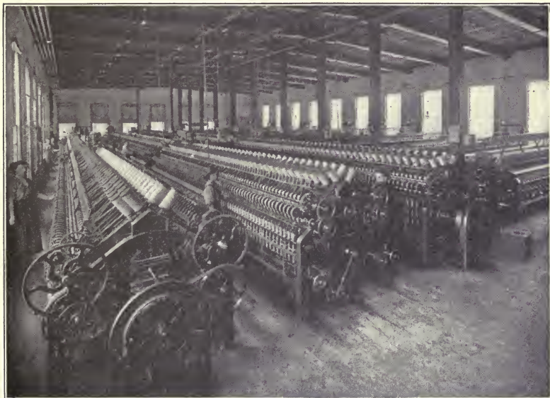
FIG. 125. — The spinning of wool into yarn.
