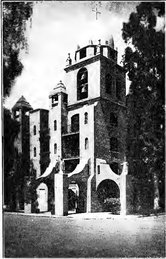
CARMEL TOWER, GLENWOOD MISSION INN
