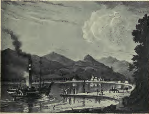
AT LOCH GOIL JETTY
