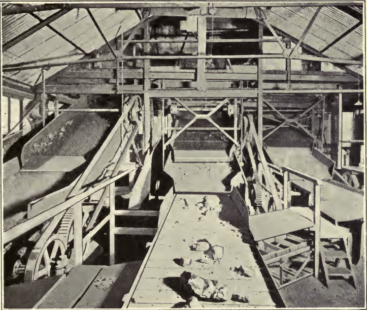
FIG. 30.—View of interior of screening shed, showing jigging shoot, screens and belts.
