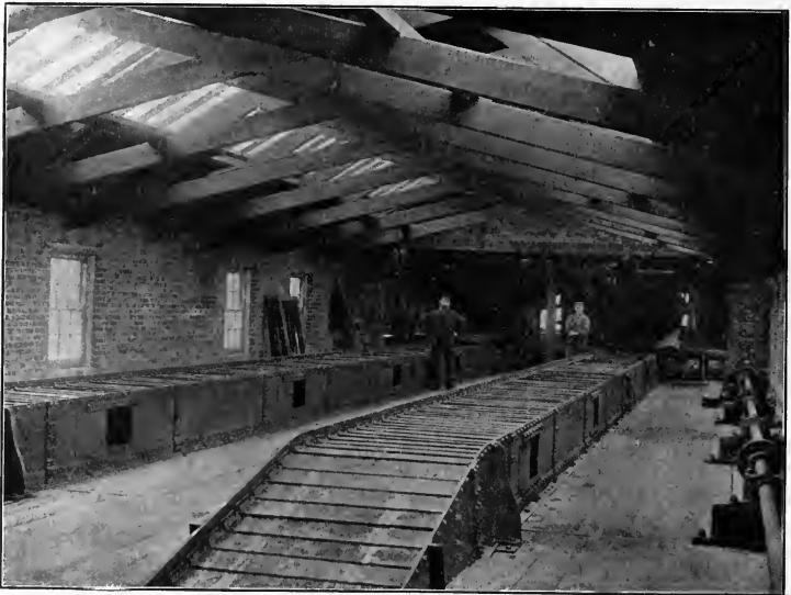
FIG. 36.—Plant constructed for the Cramlington Coal Co., Northumberland, and arranged to screen and pick 800 tons per day.
