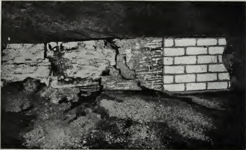
FIG. 13. Fire-seal repaired by Pyrobar
