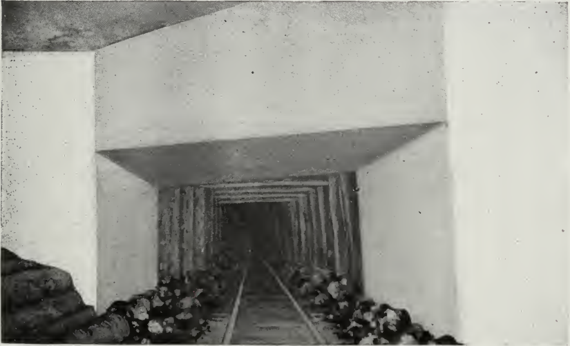
FIG. 14. Concrete overcast
