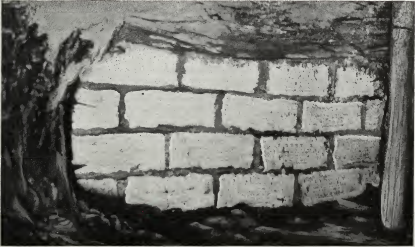
FIG. 11. Stopping built of Pyrobar block
