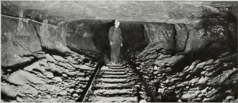
FIG. 16. Entry sixteen feet wide without timber
