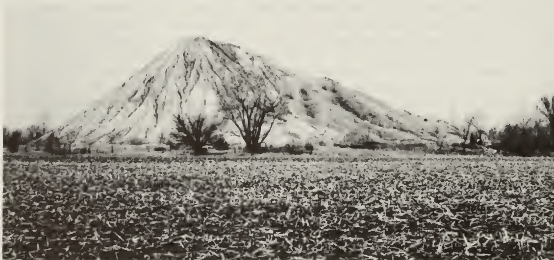
Figure 2. The mining gob pile at Rutland, La Salle County, is 112 feet high and 550 feet long. The rails ran up the longer slope on the right between the hoisting shaft and the peak.
