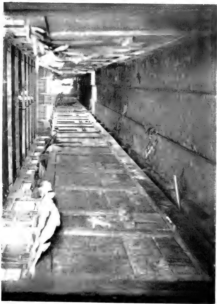
FERMENTING CHAMBERS, "AGUA IZÉ" ESTATE, SAN THOMÉ
