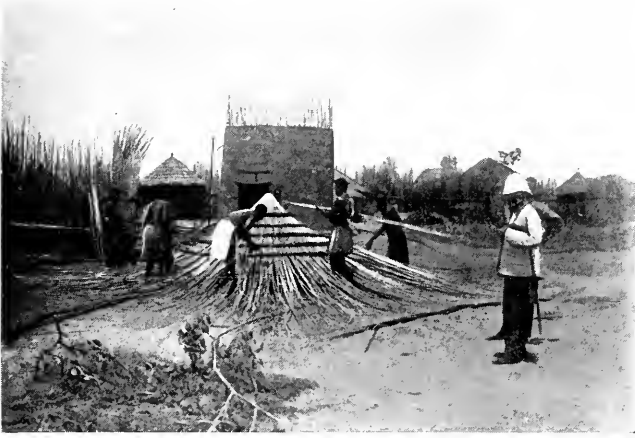
Stage I.—Raising the roof.
