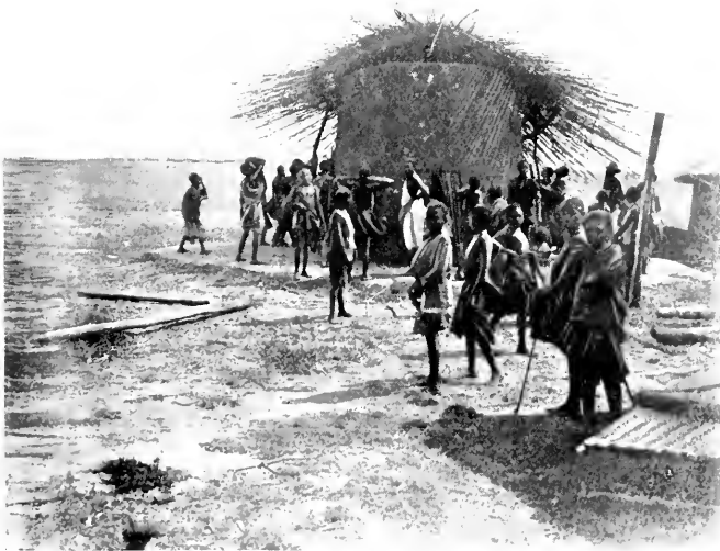
Stage II.— Putting on the roof. The school-children are much interested.
