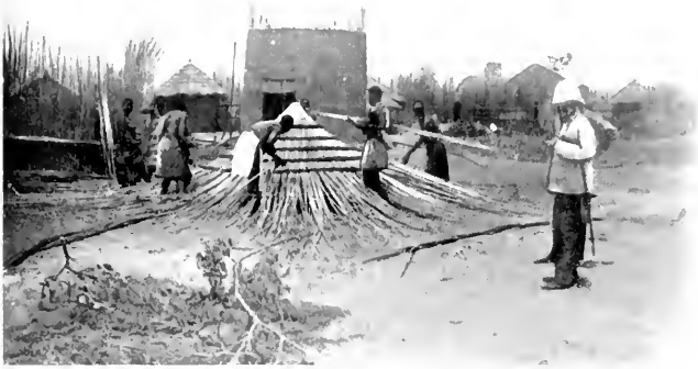
Stage I. Raising the roof.
