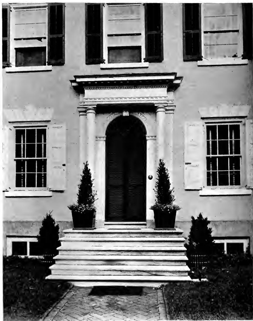
PLATE XXX. — Doorway, Doctor Denton's House, Germantown.
