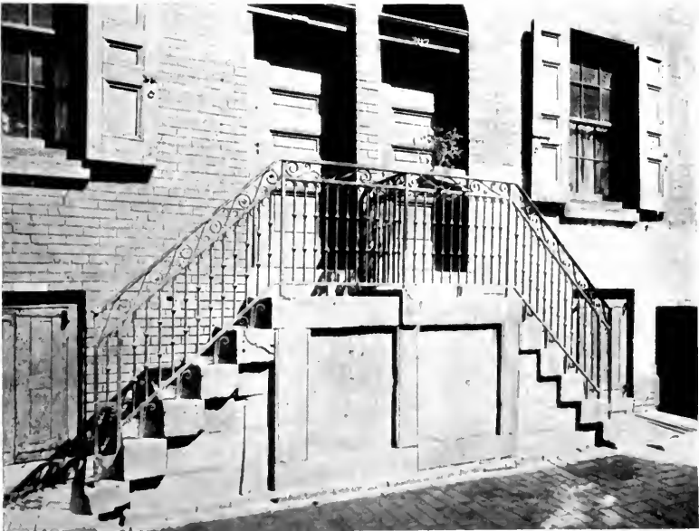
PLATE XXXVIII. — Detail of Iron Balustrade, 216 South Ninth Street; Stoop with Wing Flights, 207 La Grange Alley.
