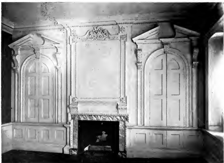
PLATE LXI. — Chimney Piece in the Hall, Stenton; Chimney Piece and Paneled Wall, Great Chamber, Mount Pleasant.
