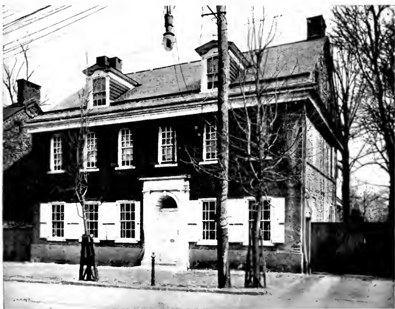
PLATE X. — Glen Fern, on Wissahickon Creek, Germantown. Erected about 1747 by Thomas Shoemaker; Grumble- thorpe, 5261 Germantown Avenue, Germantown. Erected in 1744 by John Wister.
