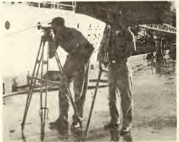
Improved harbor facilities demand more accurate tidal predictions. Two officers of the ESSA Commissioned Corps run a line of levels to tie in a tide gauge with bench marks of known elevation on the land.
