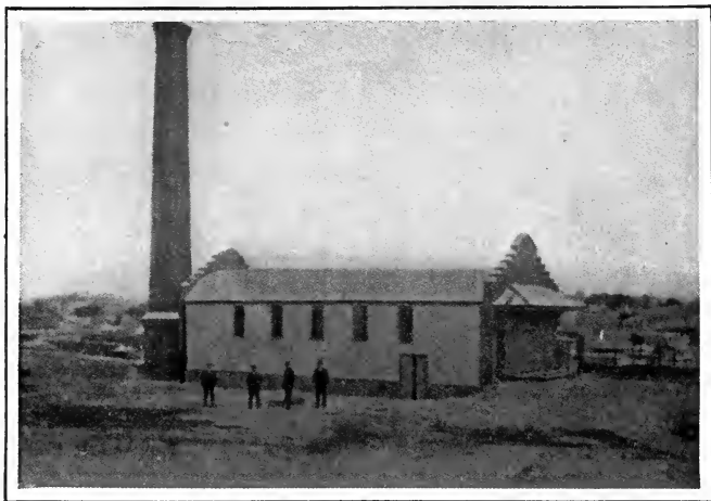
FIG. 85.—DESTRUCTOR AT ANNANDALE, AUSTRALIA.
