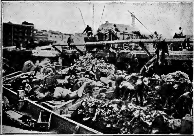
FIG. 11.—TIPPING ASHES AND RUBBISH INTO SCOWS, N. Y. CITY.
