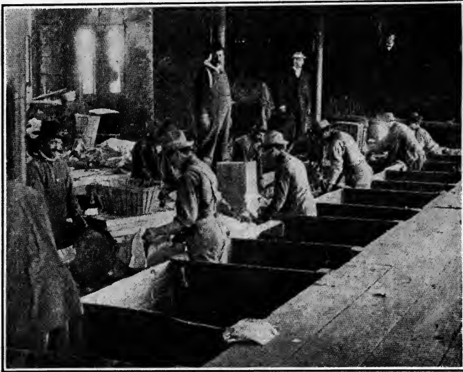
FIG. 6.—CONVEYOR AND SORTING BINS, NEW YORK STATION.
