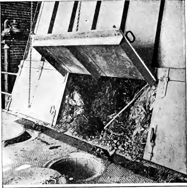
FIG. 67.—REFUSE HOPPER AND CHARGING HOLES, WESTMOUNT DESTROYER.
