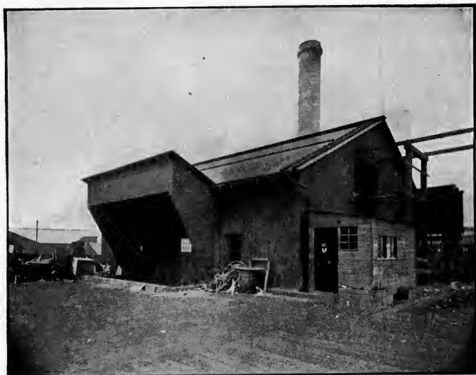
FIG. 73.—FRONT OF DESTRUCTOR PLANT, SEATTLE, WASH.
