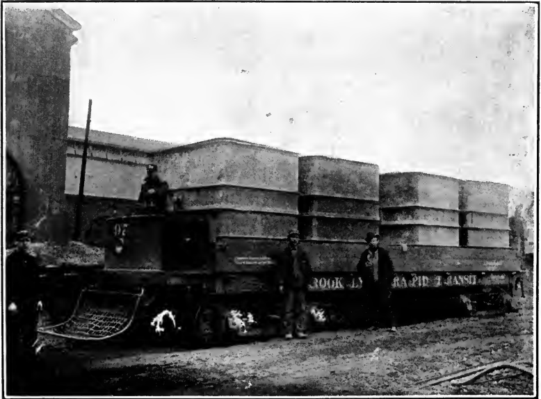
FIG. 13.—ASH BINS REMOVED BY TROLLEY, BROOKLYN.
