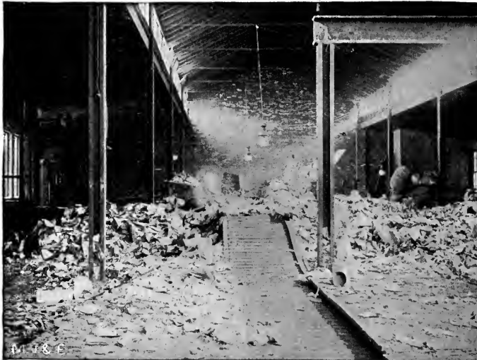
FIG. 2.—THE RECEIVING ROOM AND CONVEYOR, BOSTON.
