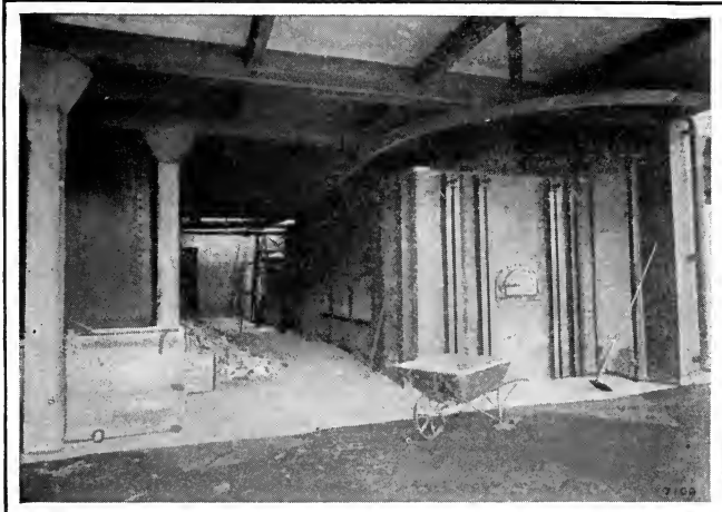
FIG. 83.—DESTRUCTOR AT STOKE-ON-TRENT, ENGLAND.
