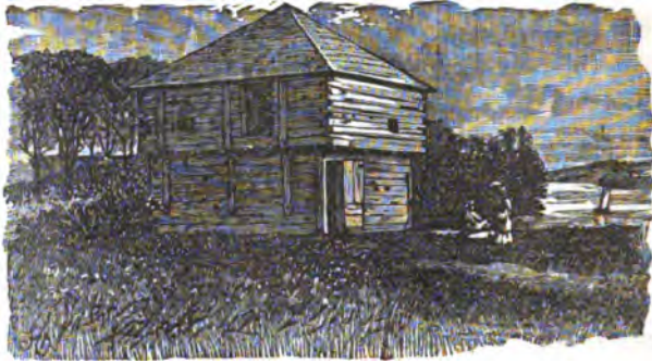
THE SOUTH FLANKER OR BLOCKHOUSE OF FORT HALIFAX, AT WINSLOW, ERECTED 1755. THE UPRIGHT PLANKS ON ONE SIDE HAVE BEEN RECENTLY PLACED THERE TO SECURE THE TIMBERS.
