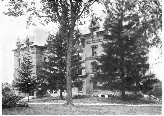
North College Dormitory
