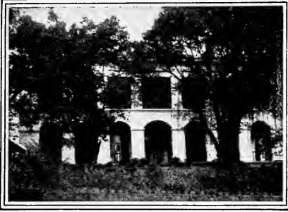
YOUNG MEN'S CHRISTIAN ASSOCIATION BUILDING AT FU-CHAU, CHINA
