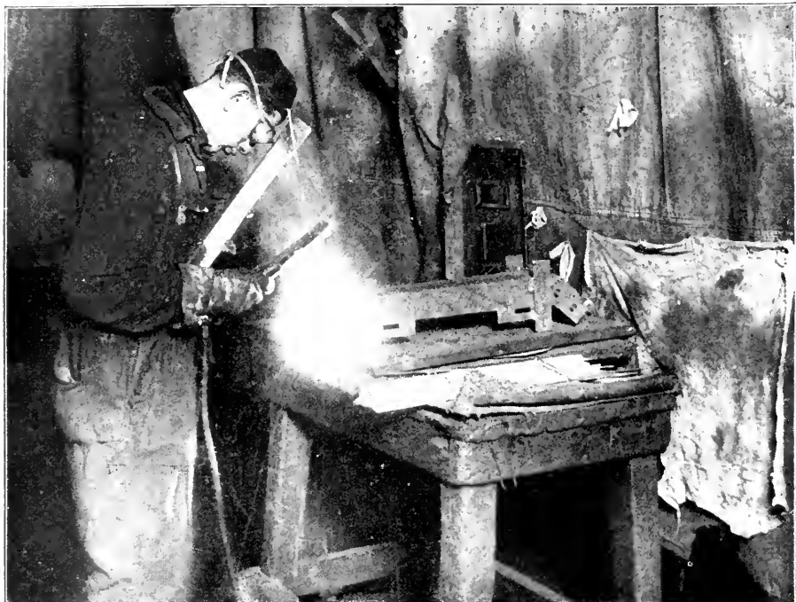
ACETYLENE WELDING ON PRESSED STEEL
