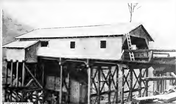
FIG. 1. LOADING STATION AT MINE
