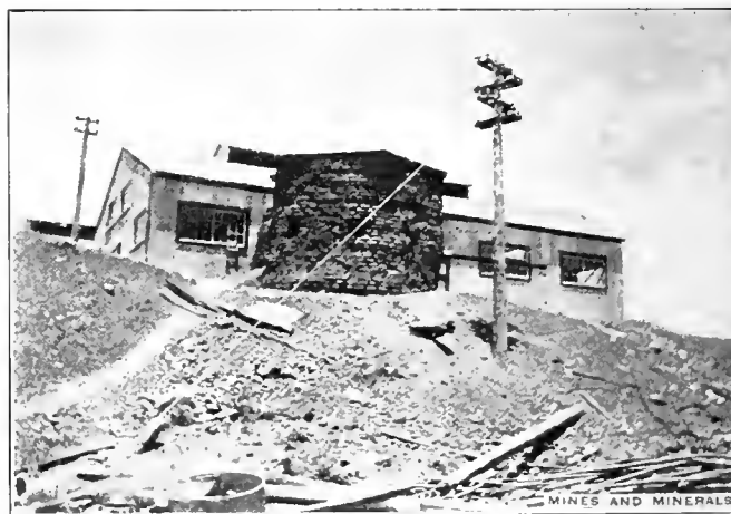
ADOBE FORT, SANTA RITA, SHOPS OF CHINO COPPER CO. IN BACKGROUND
