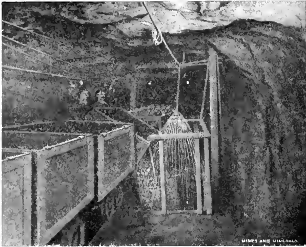
FIG. 2. SPRAYING DUST AT CHUTE
