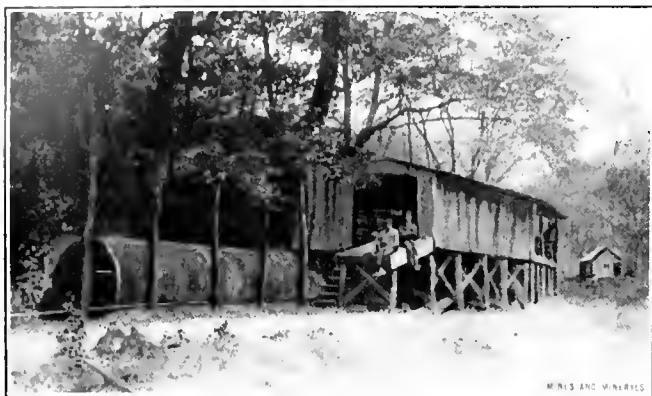
FIG. 3. STORAGE TANK, LOADING HOUSE, AND MAGNETO BUILDING
