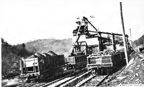
FIG. 2. LOADING CARS FROM TRAMWAY
