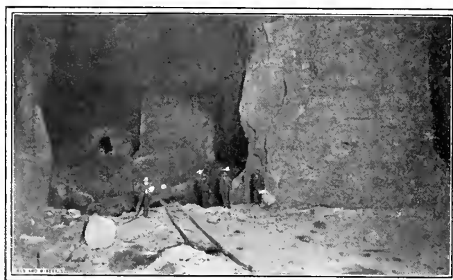
FIG. 2. PILLARS IN DISSEMINATED ZINC ORE
