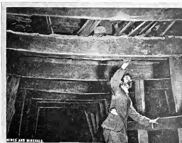
FIG. 6. SQUARED TIMBERING AT "LYE"
