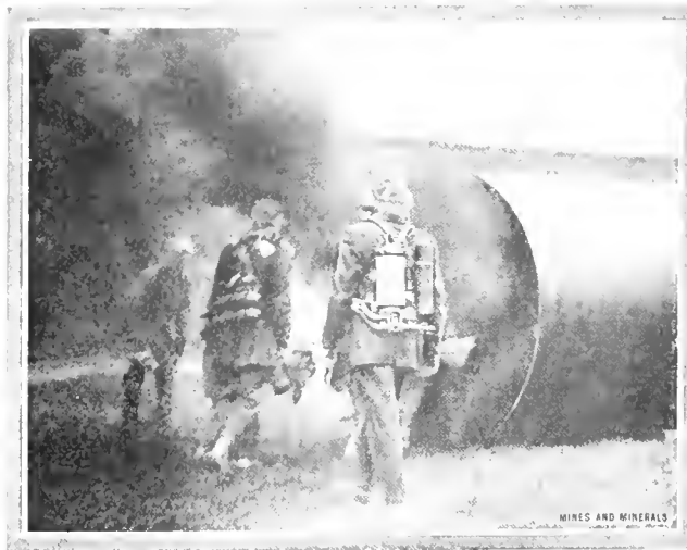
RESCUE TEAM ENTERING GALLERY AFTER EXPLOSION
