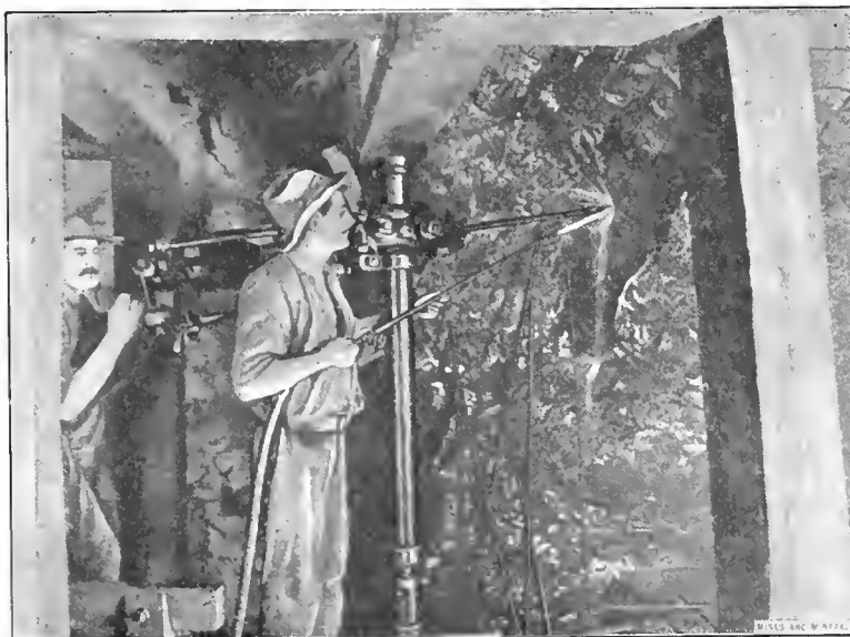
FIG. 1. SPRAYING TO PREVENT DRILL DUST
