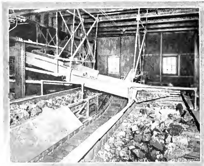
FIG. 8. SHAKING SCREEN DISCHARGING ON TO PICKING BAND
