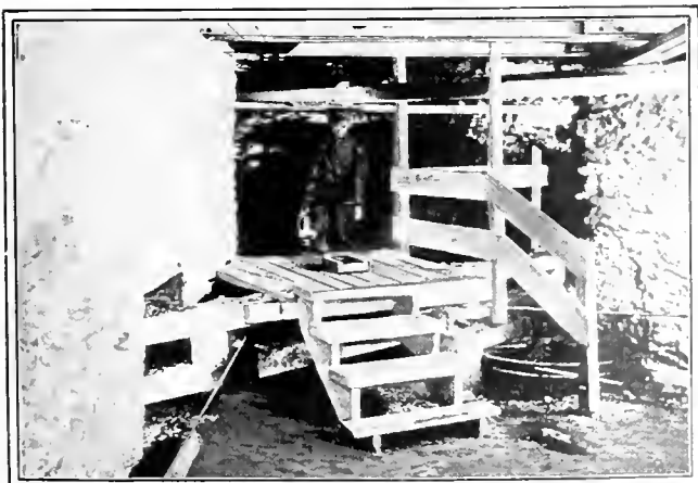
FIG. 7. CROSSING OVER HAULAGE ROPE
