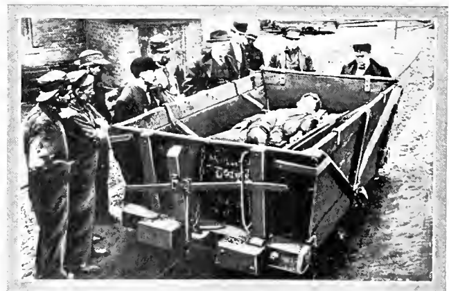
FIG. 11. HANGERS FOR STRETCHER IN MINE CAR
