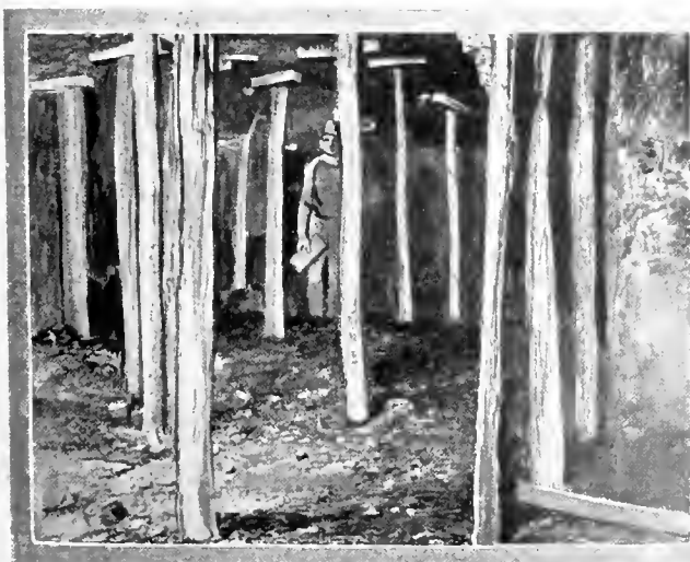
FIG. 8. TIMBER READY TO BE DRAWN IN ROOMS
