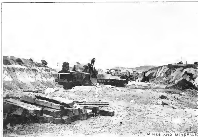
STEAM SHOVEL DIGGING ORE AFTER STRIPPING
