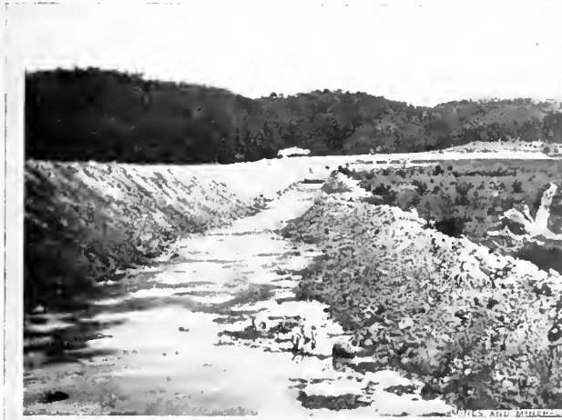
FIG. 1. SETTLING POND DAM, LOW MOOR IRON CO.
