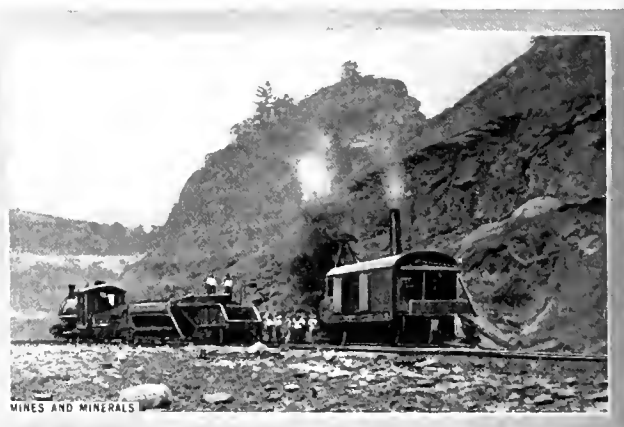
FIG. 4. STEAM SHOVEL AND ORE CAR ON THIRD STOPE
