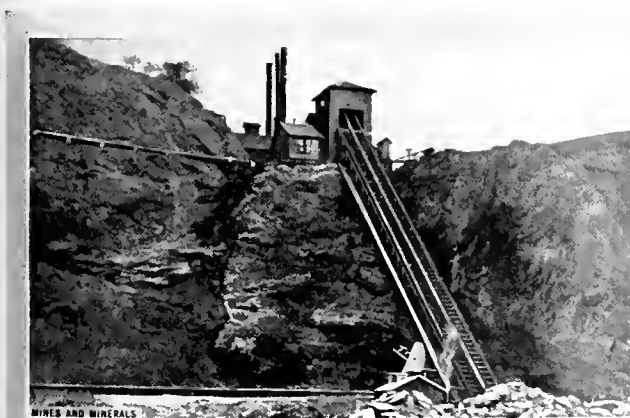
FIG. 5. EASTERN INCLINE, MIDDLE HILL MINE
