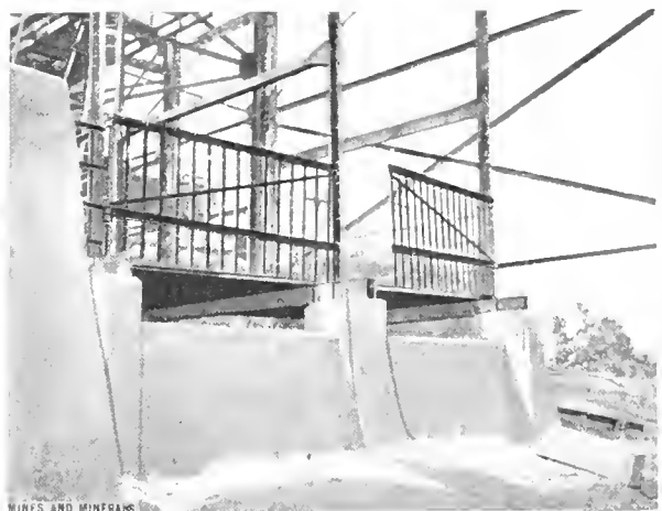
FIG. 3. TOP OF SHAFT, COMPLETED
