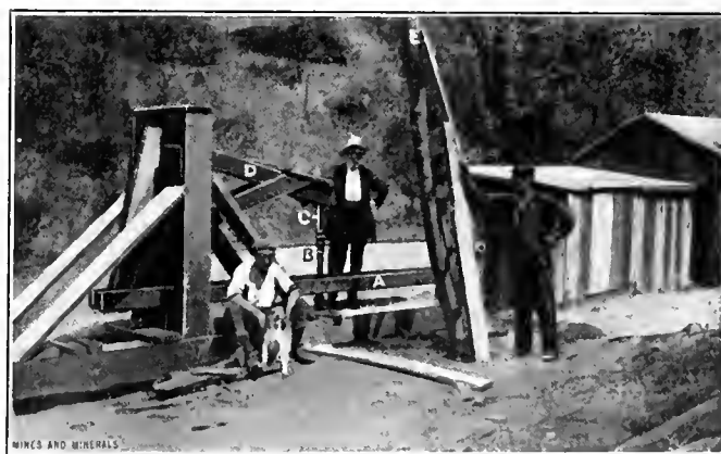
FIG. 4. HAND RIGGED PUMPING HEAD A, Connecting rod; B, Pump box; C, Pump rod; D, Lifting arm; E, Gin pole.
