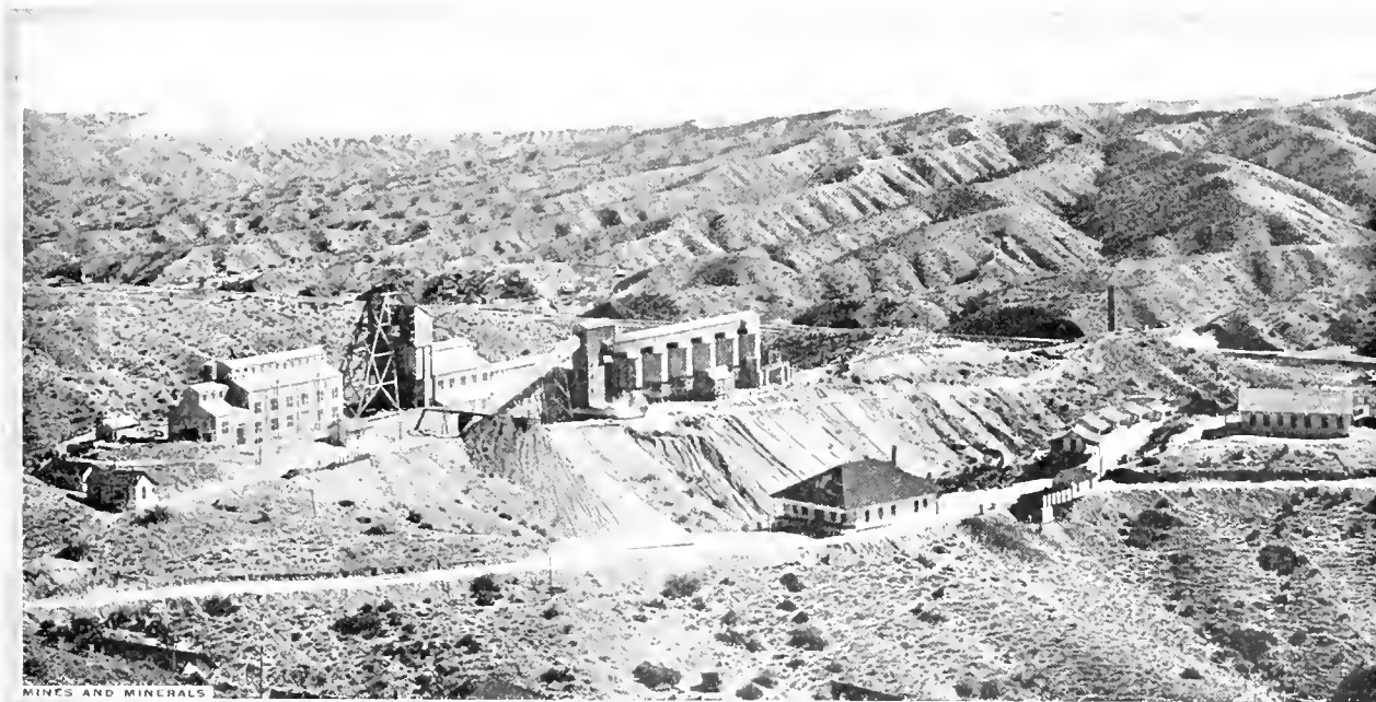
FIG. 1. HEAD-HOUSE AND BUILDINGS, MIAMI MINE
