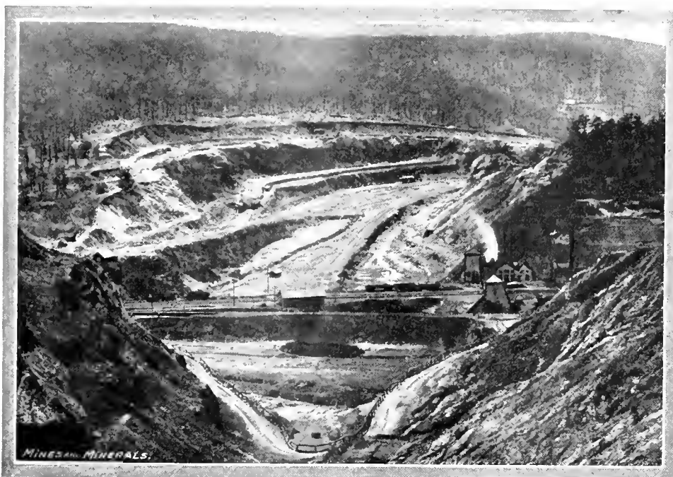
[FIG. 2. OPEN CUT WORKINGS IN MIDDLE HILL
