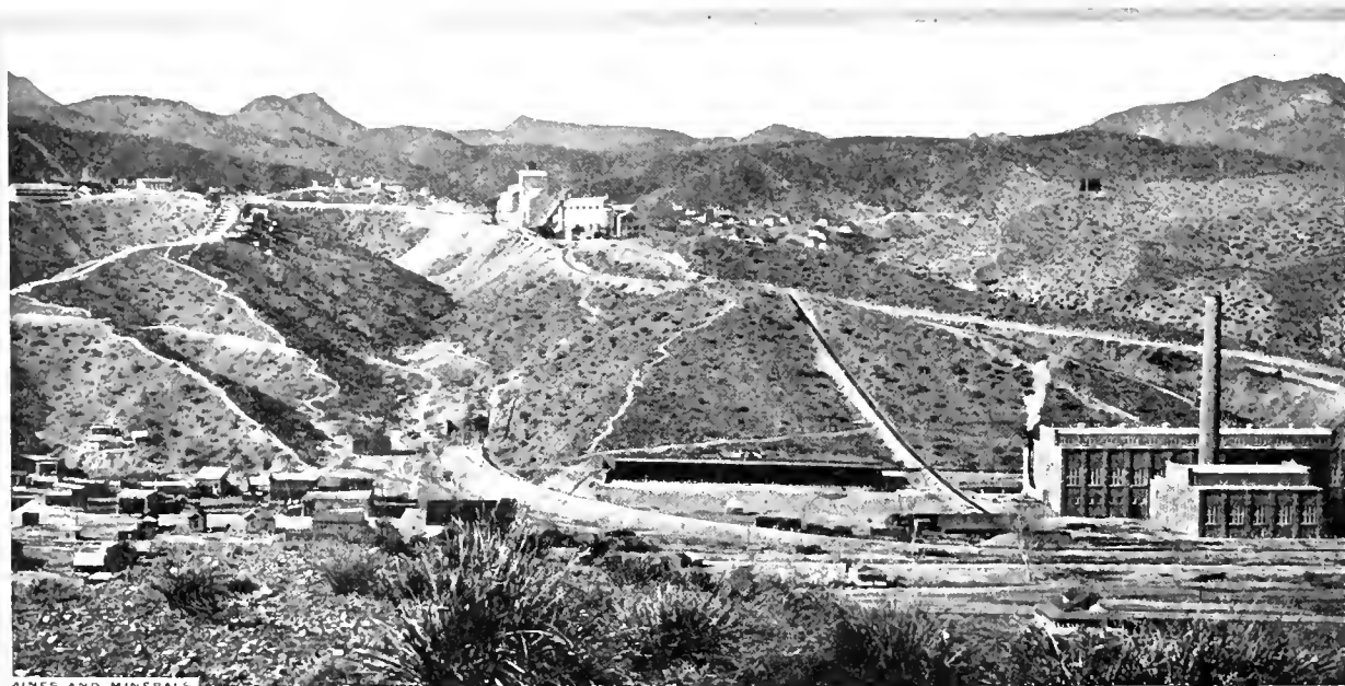
FIG. 2. VIEW LOOKING NORTH. A PORTION OF MIAMI, POWER HOUSE AT RIGHT
