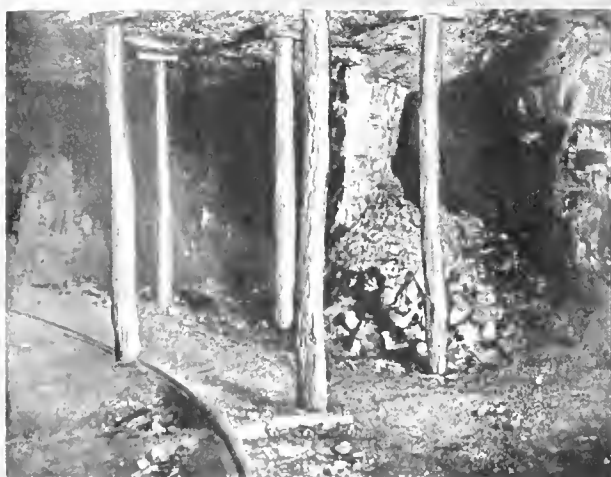
FIG. 3. LOOKING FROM ROOM TOWARD THE GOB
