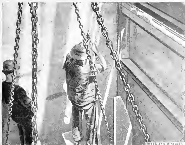
FIG. 2. DRESSING THE CONCRETE FIREPROOFING
