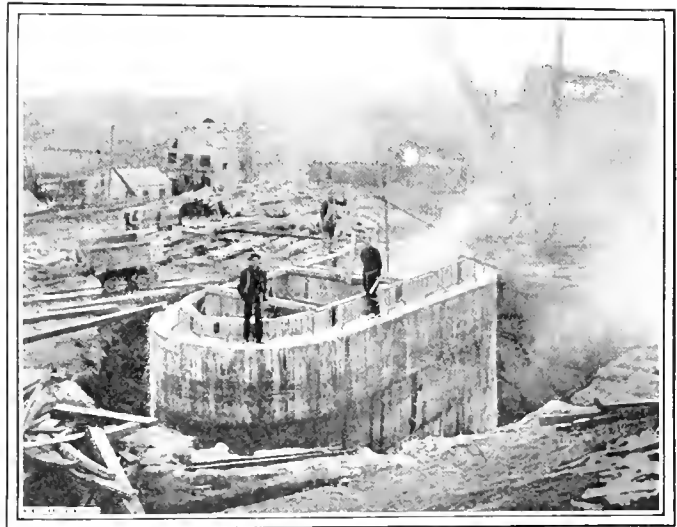
FIG. 5. VENTILATING SHAFT, CONCRETE IN PLACE BEFORE SETTLING
