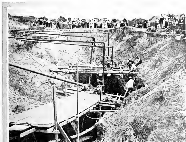
FIG. 4. RESULT OF INDISCREET DRIFTING
