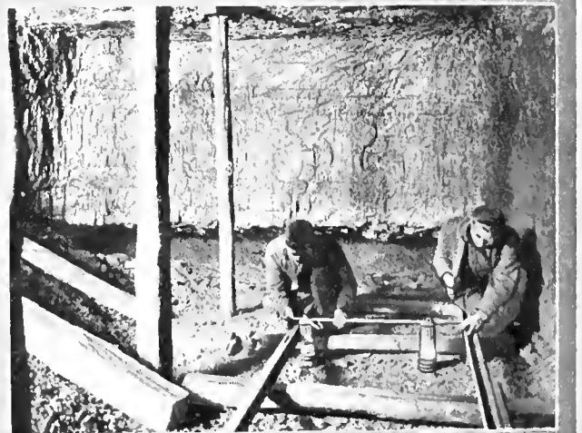
FIG. 4. LAYING TRACK
