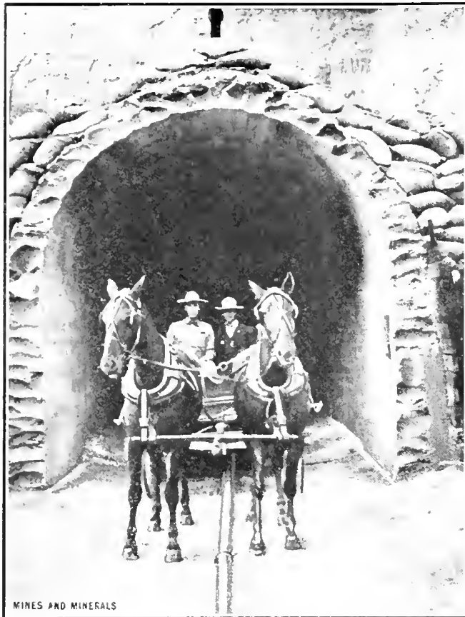
FIG. 3. PORTAL OF FINISHED TUNNEL, SAUGUS DIVISION
