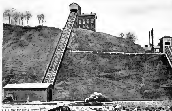
FIG. 6. NO. 2, INCLINE AND SKIP-LOADING BIN
