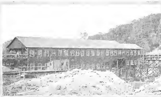
FIG. 1. STEEL TIPPLE AT NO. 2 MINE, HEILWOOD, PA.
