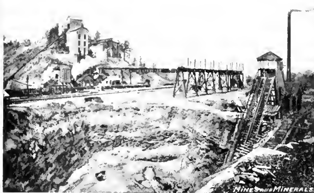
FIG. 1. CORNWALL ORE MINES No. 1 Steam Hoist to right; Robeson Hoist in center near tracks; No. 2 Hoist and Substation on hill; Ore Bin and Stock Pile in middle.
