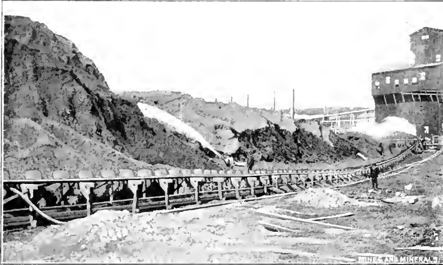
FIG. 2. HYDRAULICKING CULM TO CONVEYER LINE
