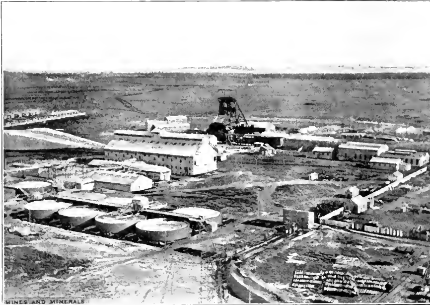
FIG. 1. SURFACE PLANT, BRAKPAN MINES, SHOWING SHAFT NO. 2
