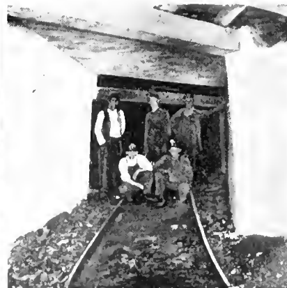
FIG. 4. PATENT LATH PLASTERED STOPPING
