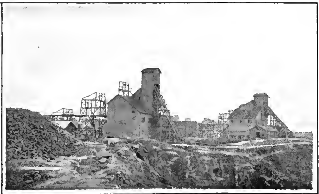
FIG. 2. SHAFT HOUSES, CREIGHTON MINE
