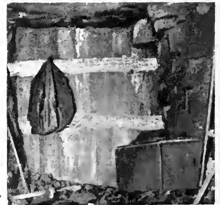
FIG. 5. BOARD STOPPING, PLASTERED
