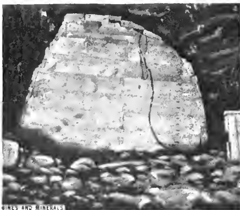
FIG. 3. SHIP-LAP PLASTERED STOPPING
