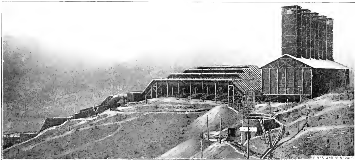
FIG. 1. BAG HOUSE AND COOLING PLANT, MAMMOTH SMELTER
