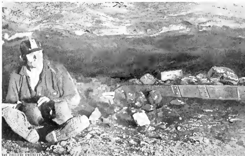
FIG. 4. CONVEYER CARRYING COAL, NEAR THE FACE
