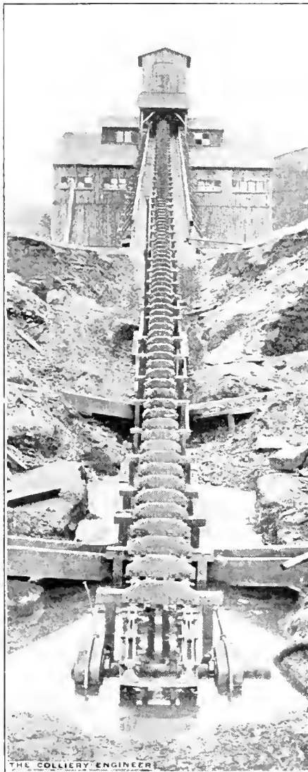
FIG. 1. SCRAPER LINE NEAR NANTICOKE, PA.
