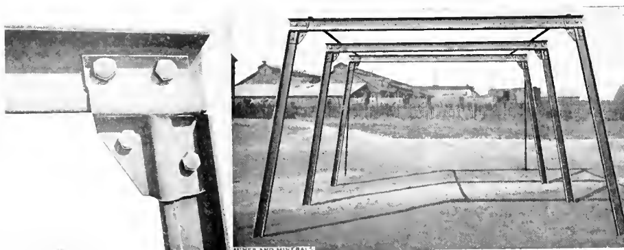
FIG. 2. STEEL MINE SUPPORT
