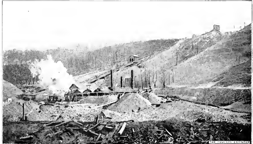
FIG. 3. LAST TWO SECTIONS OF CONVEYER LINE AT NORTH MAHANNOY COLLIERY
