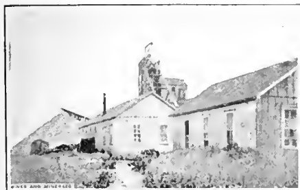
FIG. 1. ENGINE AND HOIST HOUSE, HAMILTON NO. 8 MINE
