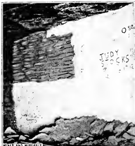
FIG. 6. SLATE STOPPING, WOOD-FIBER PLASTERED
