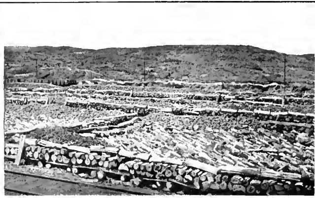
FIG. 4. WOOD PILED FOR HEAP ROASTING
