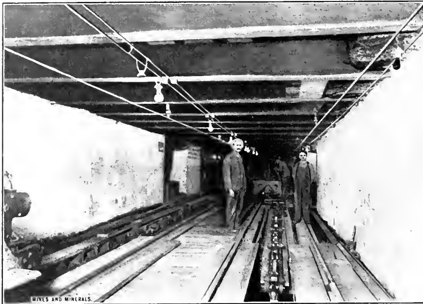
FIG. 6. PHILLIPS AUTOMATIC CAGER AND SHAFT BOTTOM
