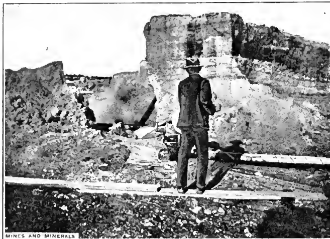
FIG. 2. BREAKING DOWN ROCK WITH HYDRAULIC NOZZLE
