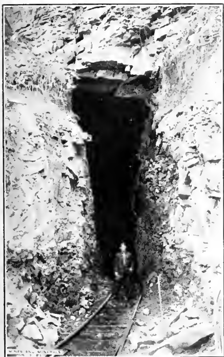
FIG. 1. OPENING AT NO. 1 MINE, ORME, TENN.
