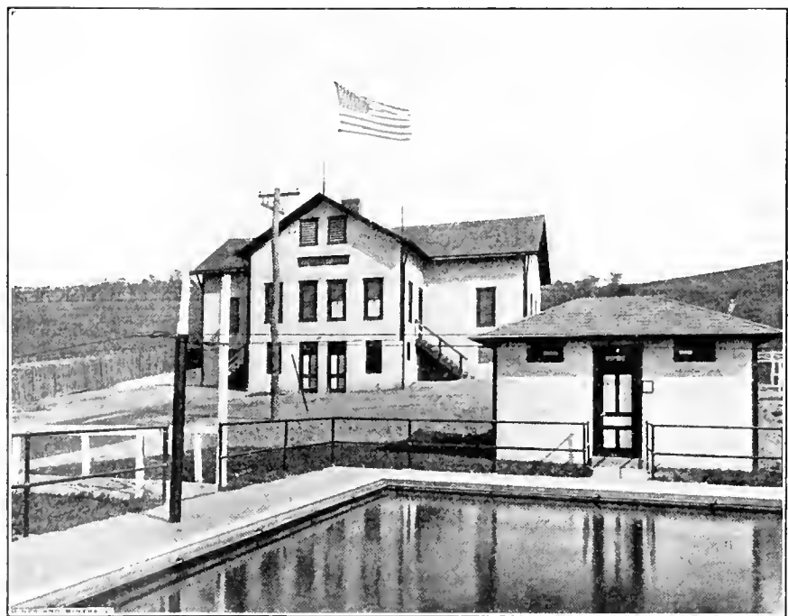
FIG 1 AMUSEMENT HALL AND SWIMMING POOL AT LEISENRING NO. 1
