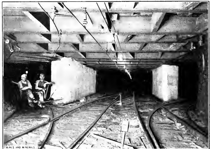
FIG. 8. TIMBERING AND CONCRETE WALLS AT TRACK INTERSECTION
