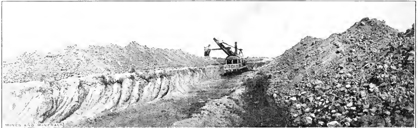
STRIPPING COAL WITH STEAM SHOVEL IN KANSAS
