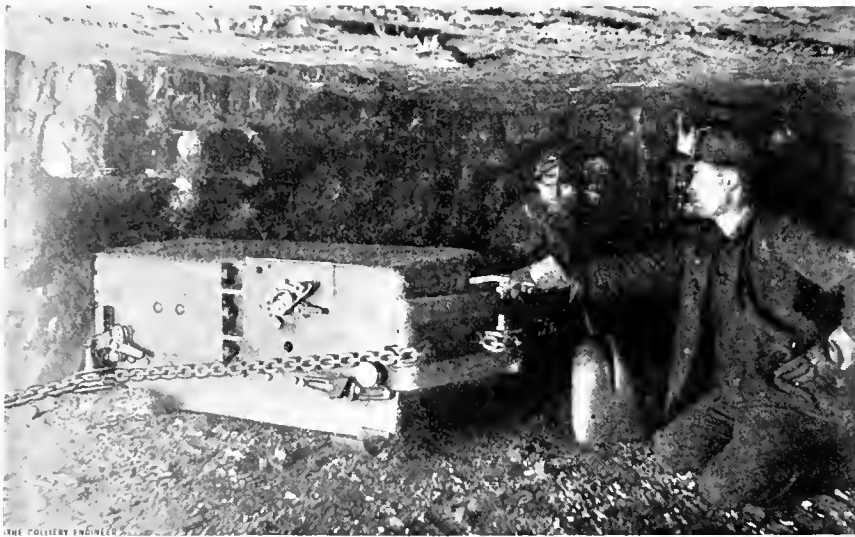
FIG. 3. SHORT-WALL MACHINE IN A 4 FT. ANTHRACITE SEAM
