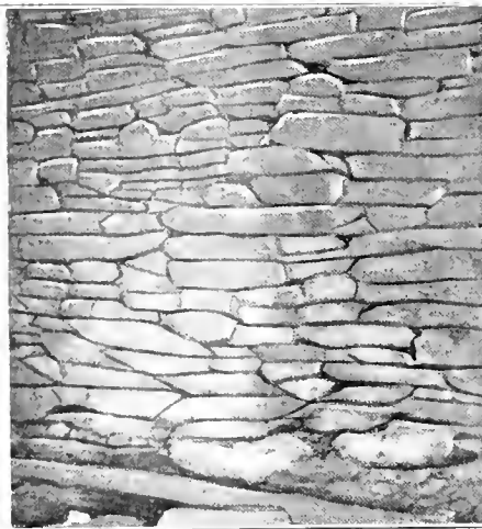
FIG. 7. SLATE STOPPING NOT PLASTERED
