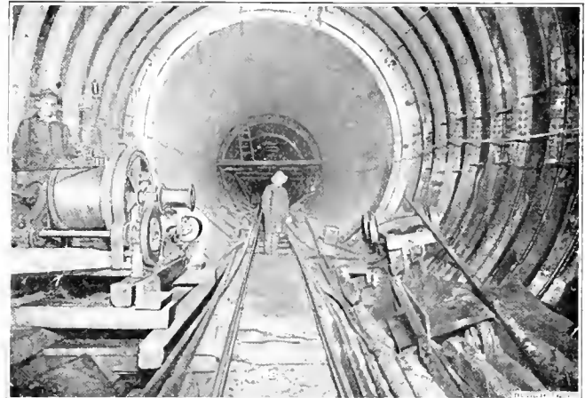
FIG. 2. RONDOUT TUNNEL, SHOWING CONCRETE AND STEEL LINING
