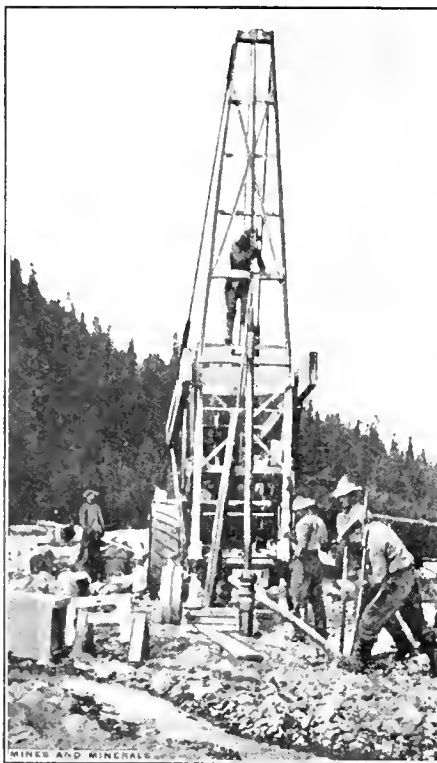
FIG. 1. DRIVING CASING
