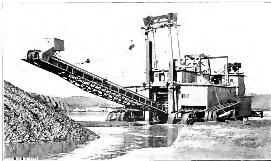
FIG. 2. DREDGE, SHOWING TAILING STACKER AND DISCHARGE LAUNDER
