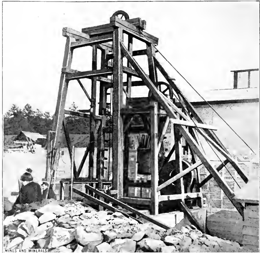
FIG 1 TEMPORARY SHAFT HEAD
