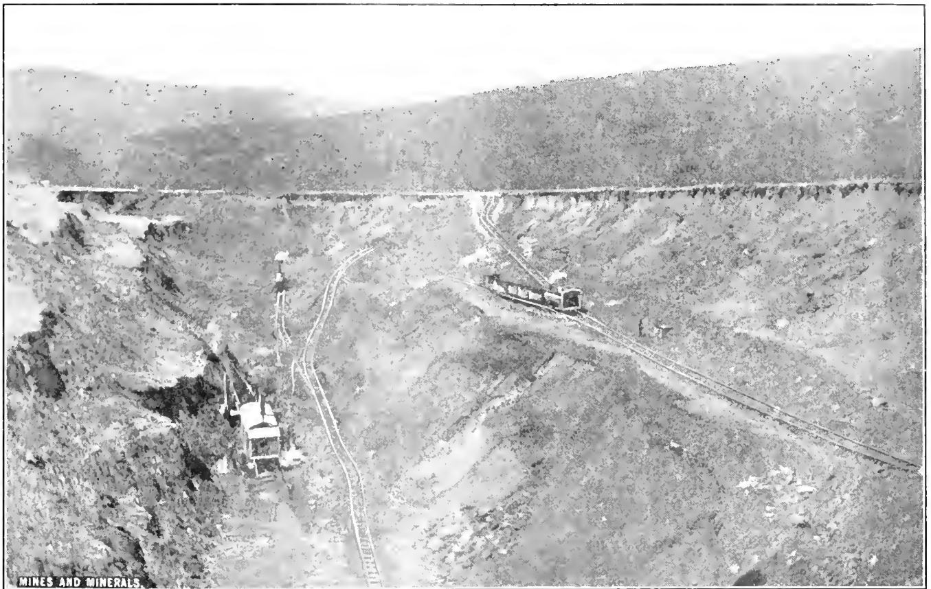
FIG. 1. ANTHRACITE STRIPPING AT DERRINGER, PA.
