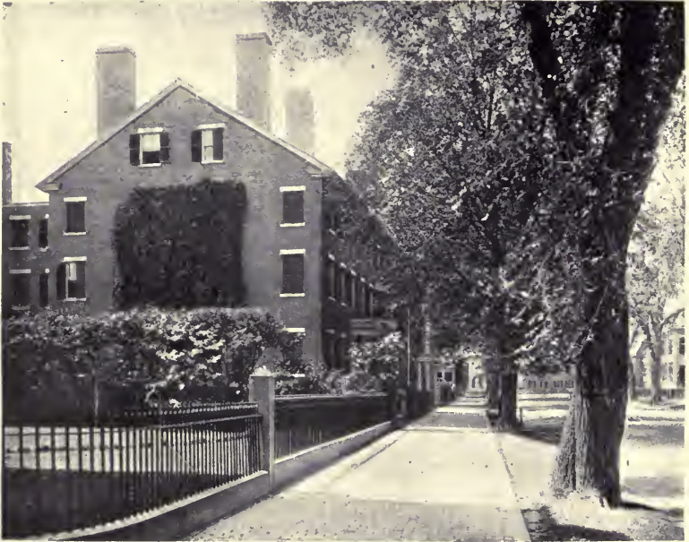
PLATE XLIII. — Hoffman-Simpson House, 26 Chestnut Street. Erected about 1827; Allen-Osgood-Huntington Houses, 31, 33 and 35 Chestnut Street. Erected about 1825.
