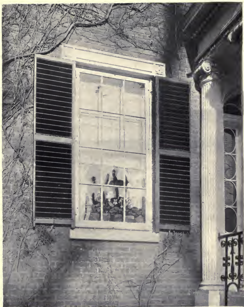
PLATE LXII. — Hoffman-Simpson Window, 26 Chestnut Street. Erected 1810.
