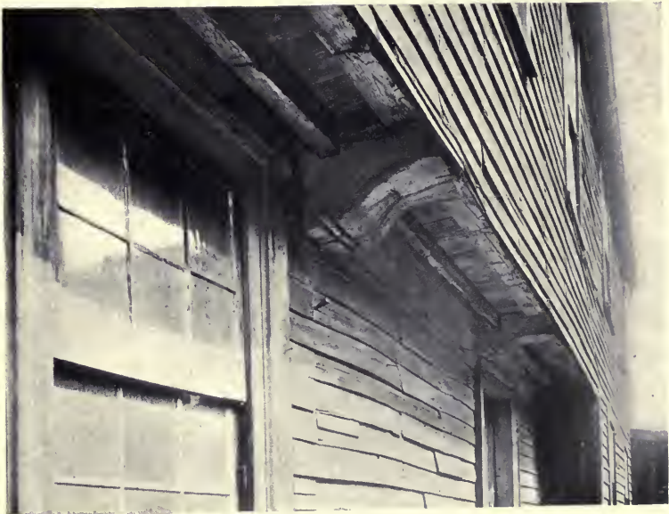
PLATE X. — The Old Bakery, formerly at 25 Washington Street. Erected 1683; Detail of Old Bakery Overhang.
