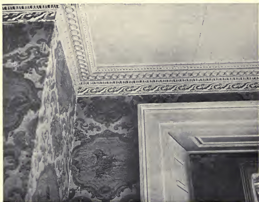
PLATE LXX. — East Front Chamber, Pierce-Johonnot-Nichols House. Finished 1801; Plaster Cornice and Frieze, Derby-Crowninshield- Rogers House. Erected 1800.
