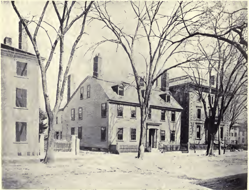
PLATE XV. — John Waters House, 5 Mason Street. Erected 1800; Wheatland House, 374 Essex Street. Erected before 1773.
