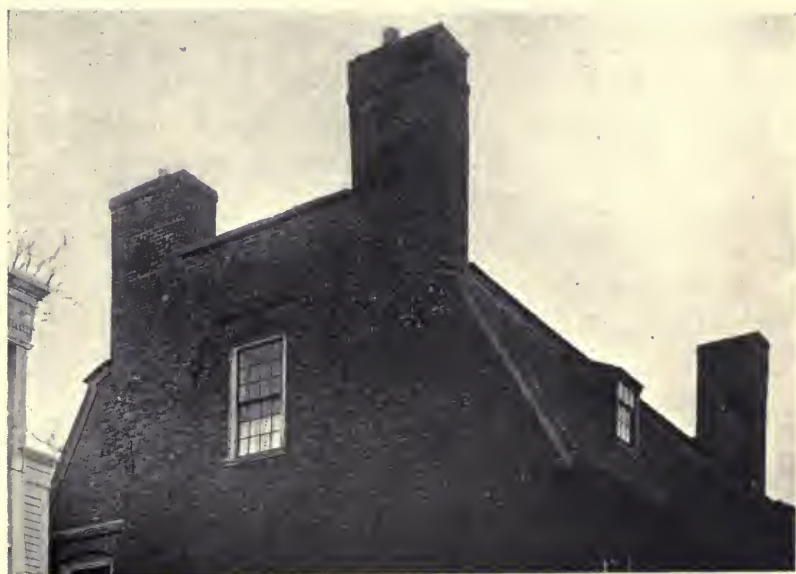
PLATE XXIV.—Richard Derby House, 168 Derby Street. Erected 1761; Gambrel Gable and Chimneys, Richard Derby House.
