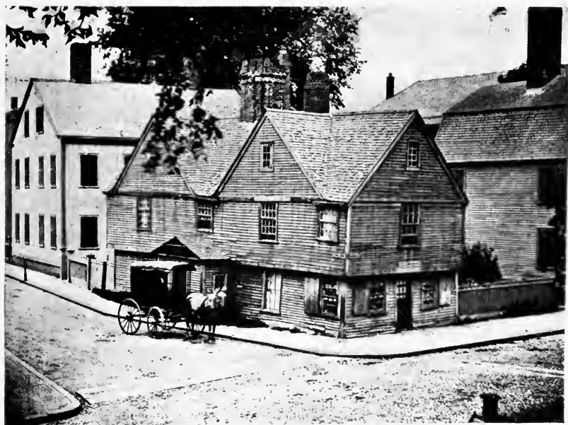
PLATE VI. — Philip English House. Erected in 1685. Razed 1833; Lewis Hunt House. Erected about 1698. Razed 1863.
