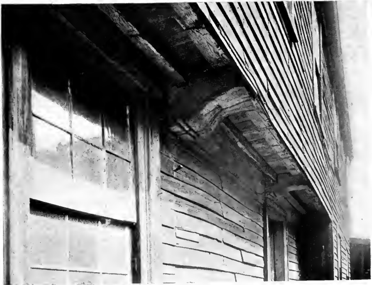
PLATE X. — The Old Bakery, formerly at 25 Washington Street. Erected 1683; Detail of Old Bakery Overhang.
