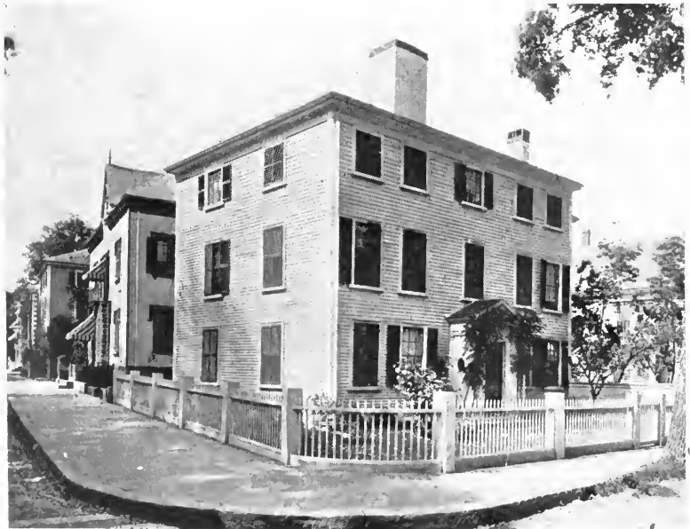
PLATE XXIX. — Captain Edward Allen House, 125 Derby Street. Erected 1780; Briggs-Whipple House, 38 Forrester Street. Erected about 1800.
