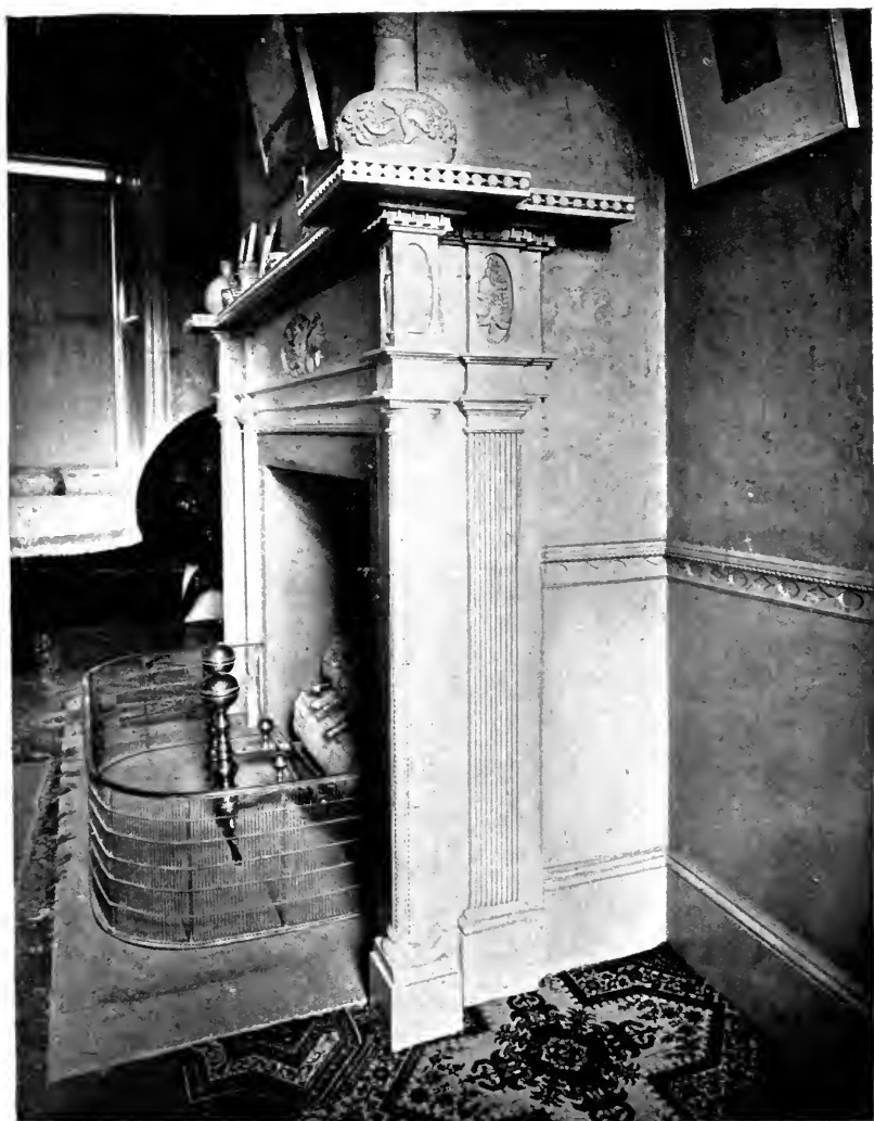
PLATE CII.—Detail of Mantel in the Kimball House.
