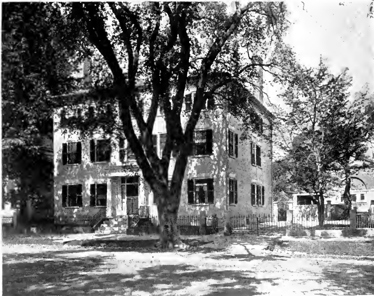
PLATE XXXIX.—Peabody-Silsbee House, 360 Essex Street. Erected 1797; Hodges-Peele-West House, 12 Chestnut Street. Erected 1804.
