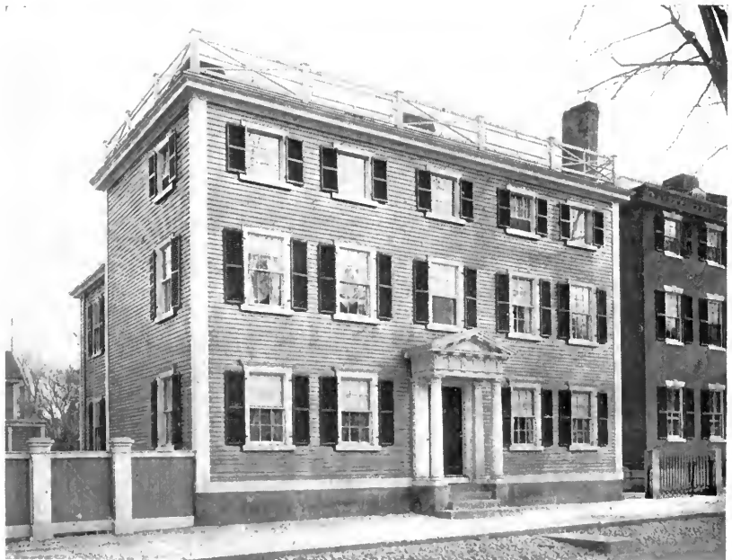
PLATE XXXI. — Timothy Orne House, 266 Essex Street. Erected 1761; Peabody-Rantoul House, 19 Chestnut Street. Erected 1810.
