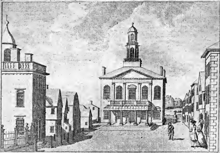
View of the COURT HOUSE, in Salem, Massachusetts.
