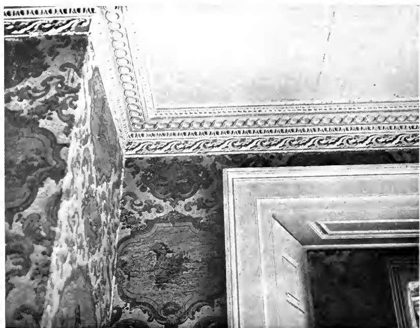
PLATE LXX. — East Front Chamber, Pierce-Johonnot-Nichols House. Finished 1801; Plaster Cornice and Frieze, Derby-Crowninshield-Rogers House. Erected 1800.
