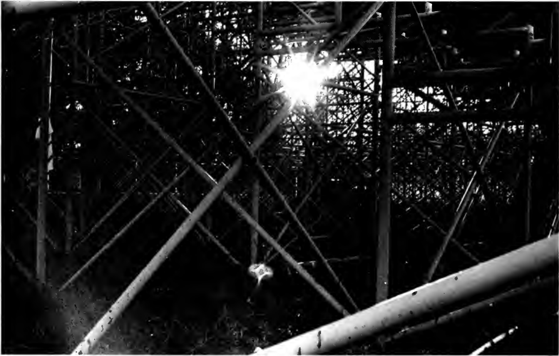
Highlighted by the setting sun, a maze of interwoven pipes supports the bleachers in the end zones
