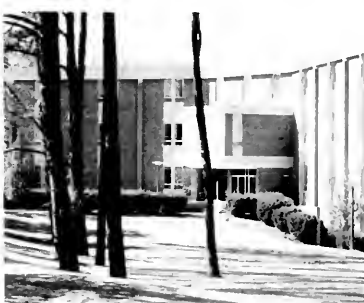
Housing a health hazard, Morton Hall is one of several academic buildings sprayed with asbestos. Some professors based in Millington and Morton refused to teach in the contaminated buildings. — Photo by Ben Wood
