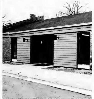
Located across from the quonset huts behind the Campus Center, the new police station was sorely needed. The old "station" was designed for a campus security force, not a full police department. The new facility boasts showers, a kitchen, and a detainment cell. — Photo by Mark Beavers.
