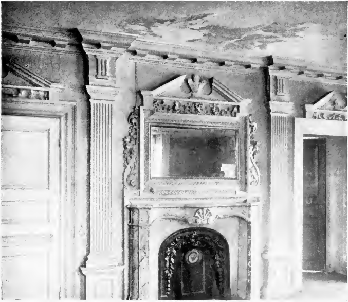
MANTEL AND MIRROR OF SECOND-STORY-FRONT ROOM IN PHILIPPE MANOR-HOUSE.
