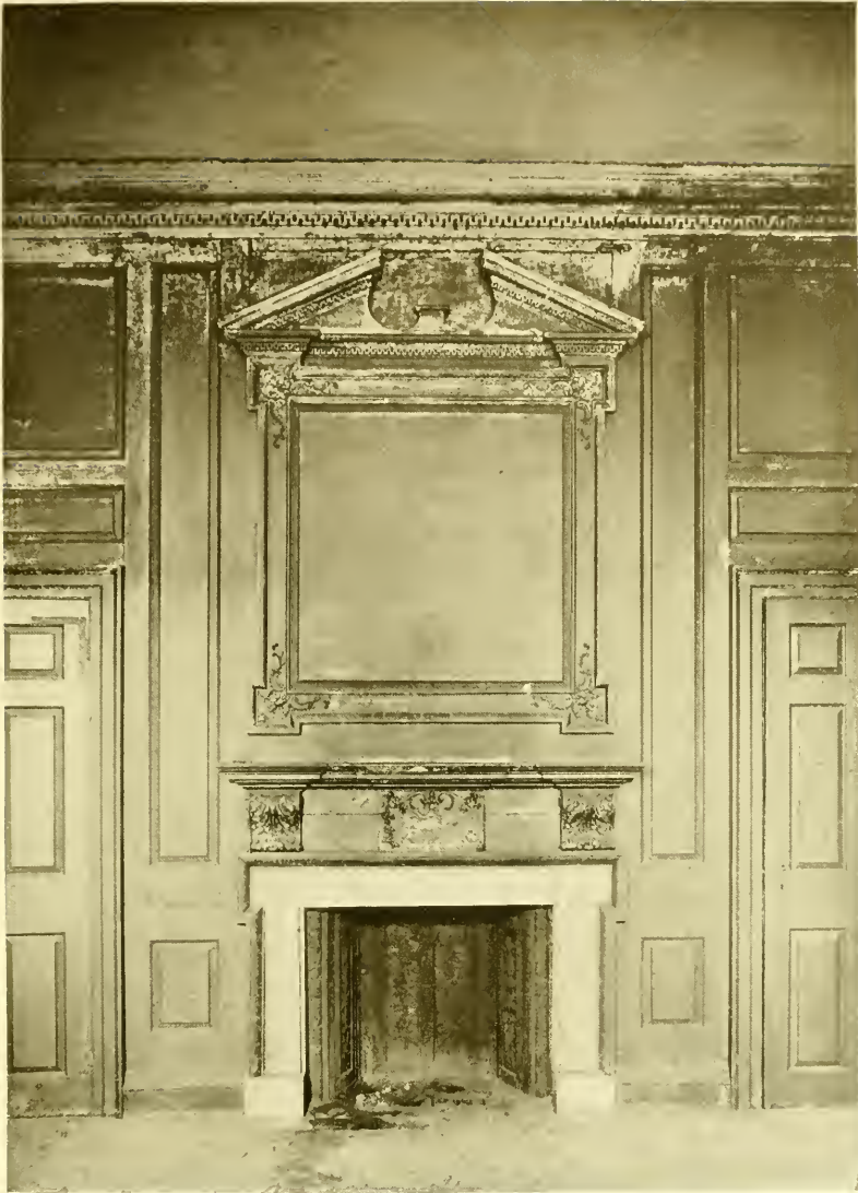
FIREPLACE AND OVER-MANTEL IN BEDCHAMBER OF POWEL HOUSE
