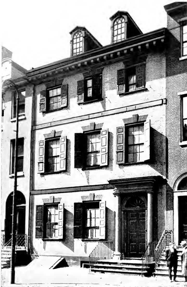
POWEL HOUSE, NUMBER 244 SOUTH THIRD STREET Built c. 1762.
