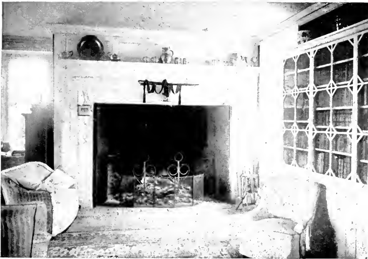
LIVING ROOM AT WAYNESBOROUGH
