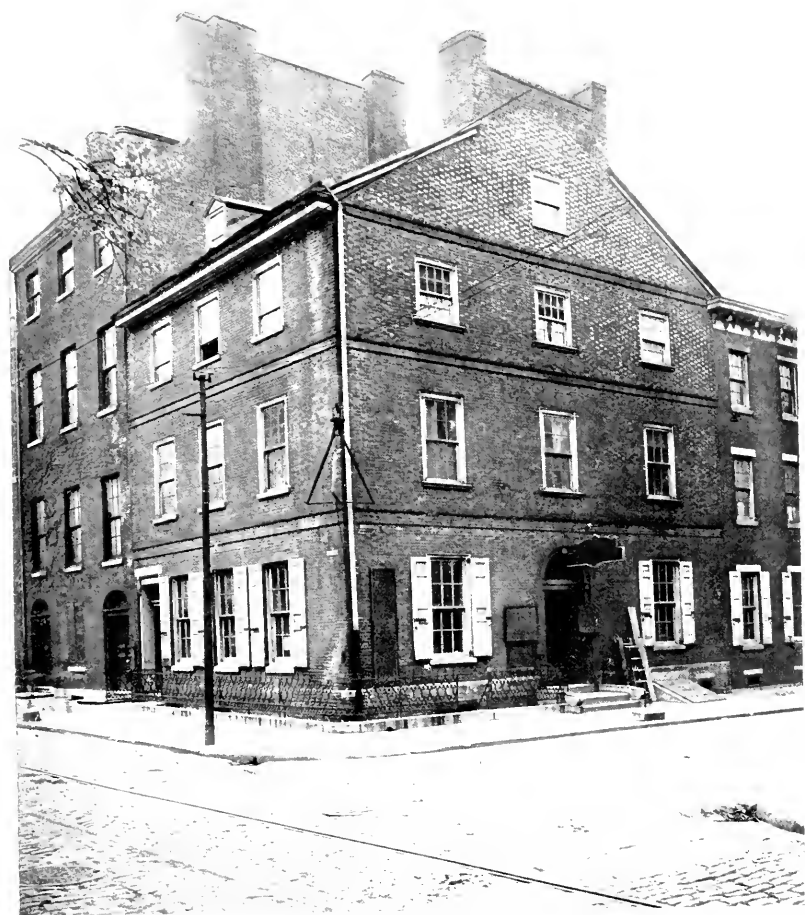
WISTAR HOUSE, SOUTHWEST CORNER OF FOURTH AND PRUNE (LOCUST) STREETS. CADWALADER HOUSE TO THE LEFT
