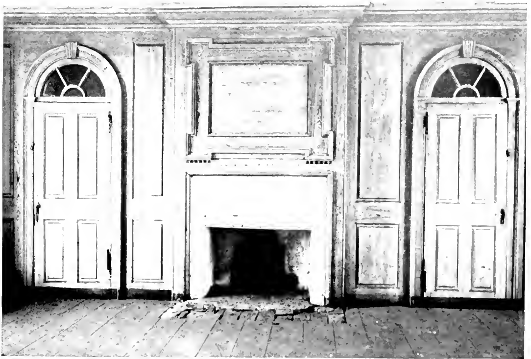
GREAT CHAMBER ON SECOND FLOOR AT GRAEME PARK
