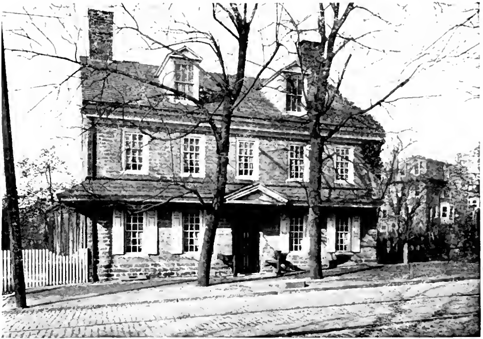
JOHNSON HOUSE, 6305 GERMANTOWN ROAD Built by John Johnson, 1760
