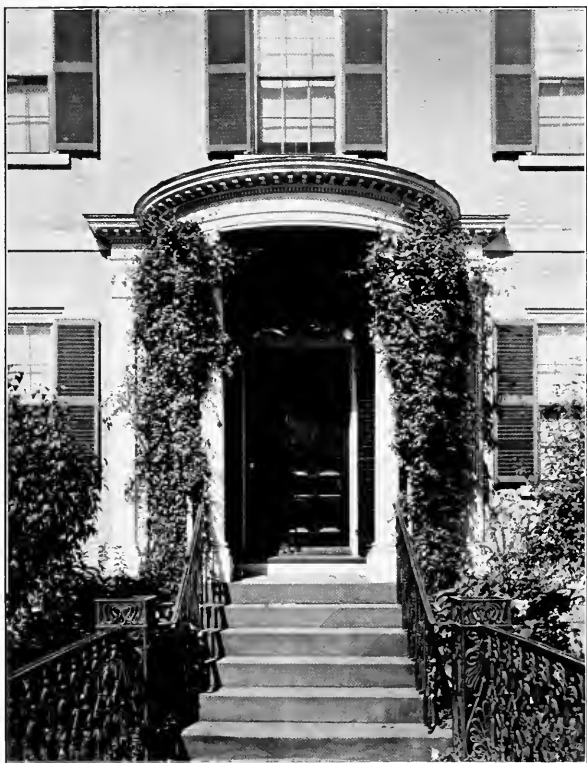
PLATE XI. — Gardner House Doorway, 1804.
