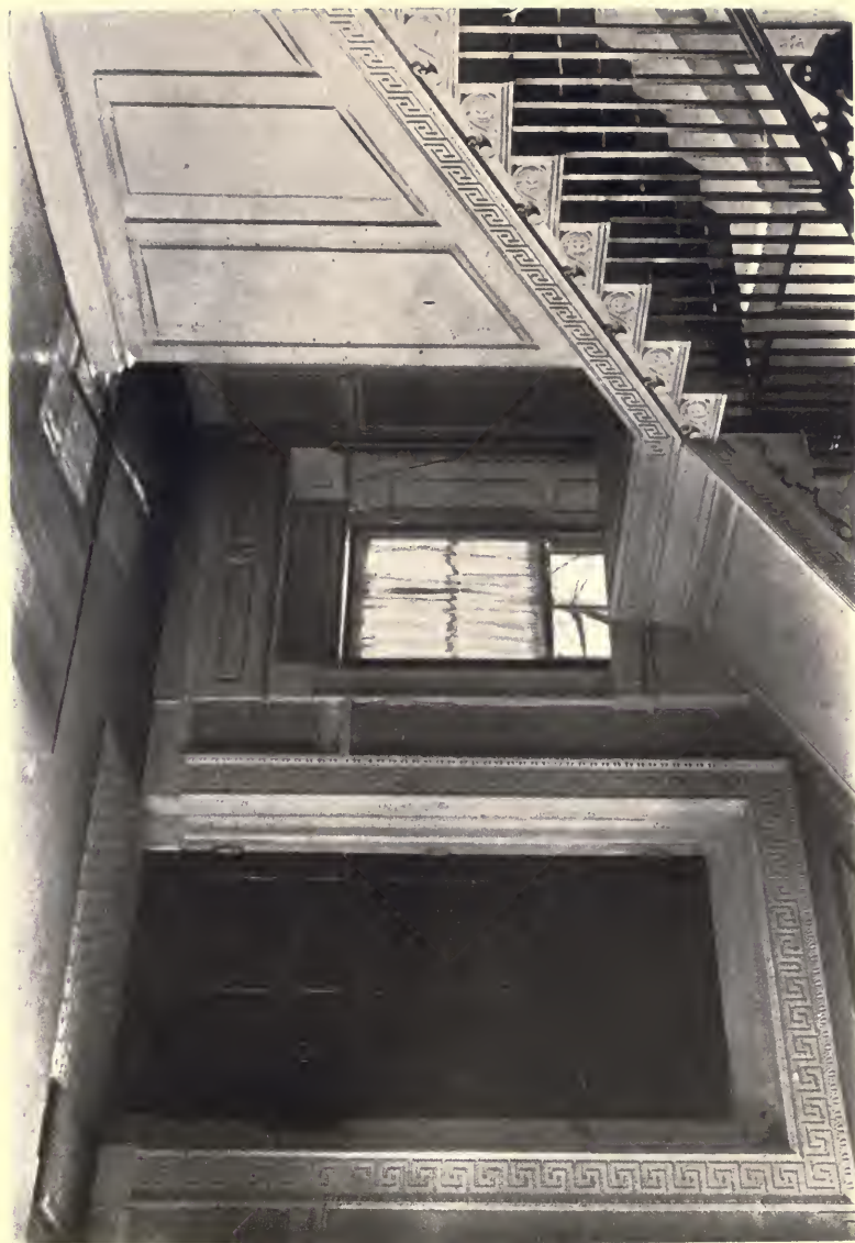
ENTRANCE HALL OF SCOTT HOUSE
