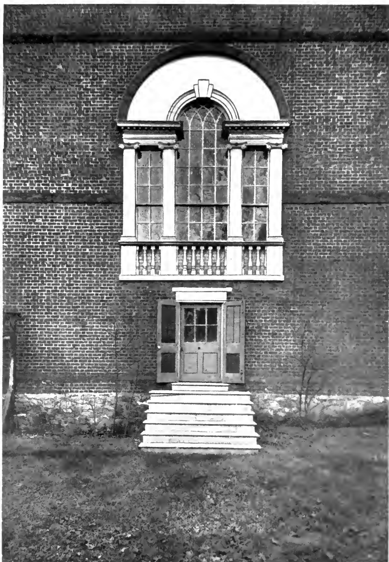
PALLADIAN WINDOW IN CHASE HOUSE
