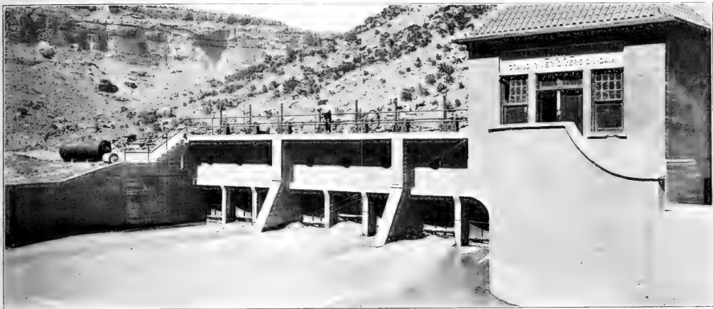
Grand Valley Project. Gates in Grand River Dam turning the water into the high line canal. U. S. Reclamation Service
