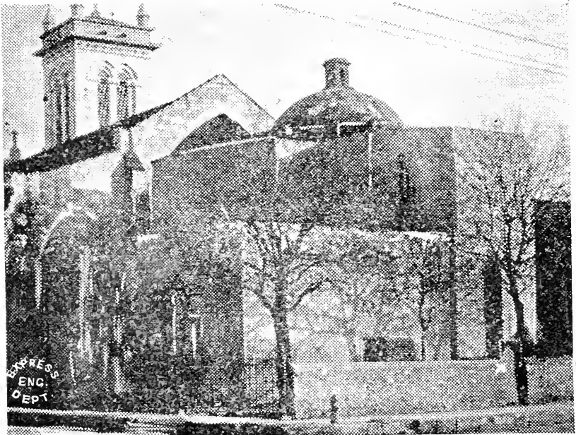
ORIGINAL MORESCUE DOMED BUILDING FORMING REAR OF SAN FERNANDO CATHEDRAL ON MILITARY PLAZA. IT IS INTACT TODAY.
