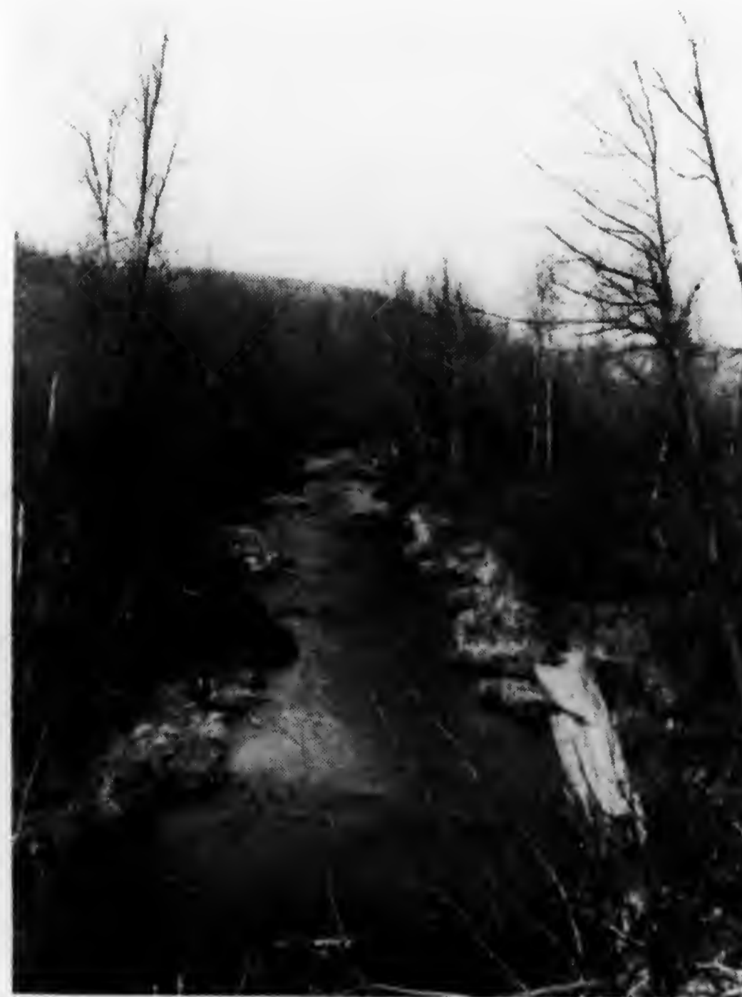
BEAR CREEK Open Section Being Improved.
