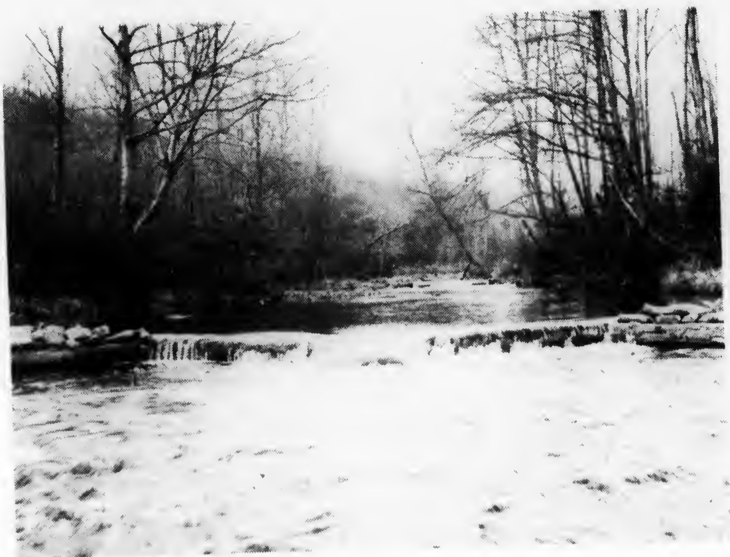
BEAR CREEK DAM No. 33
