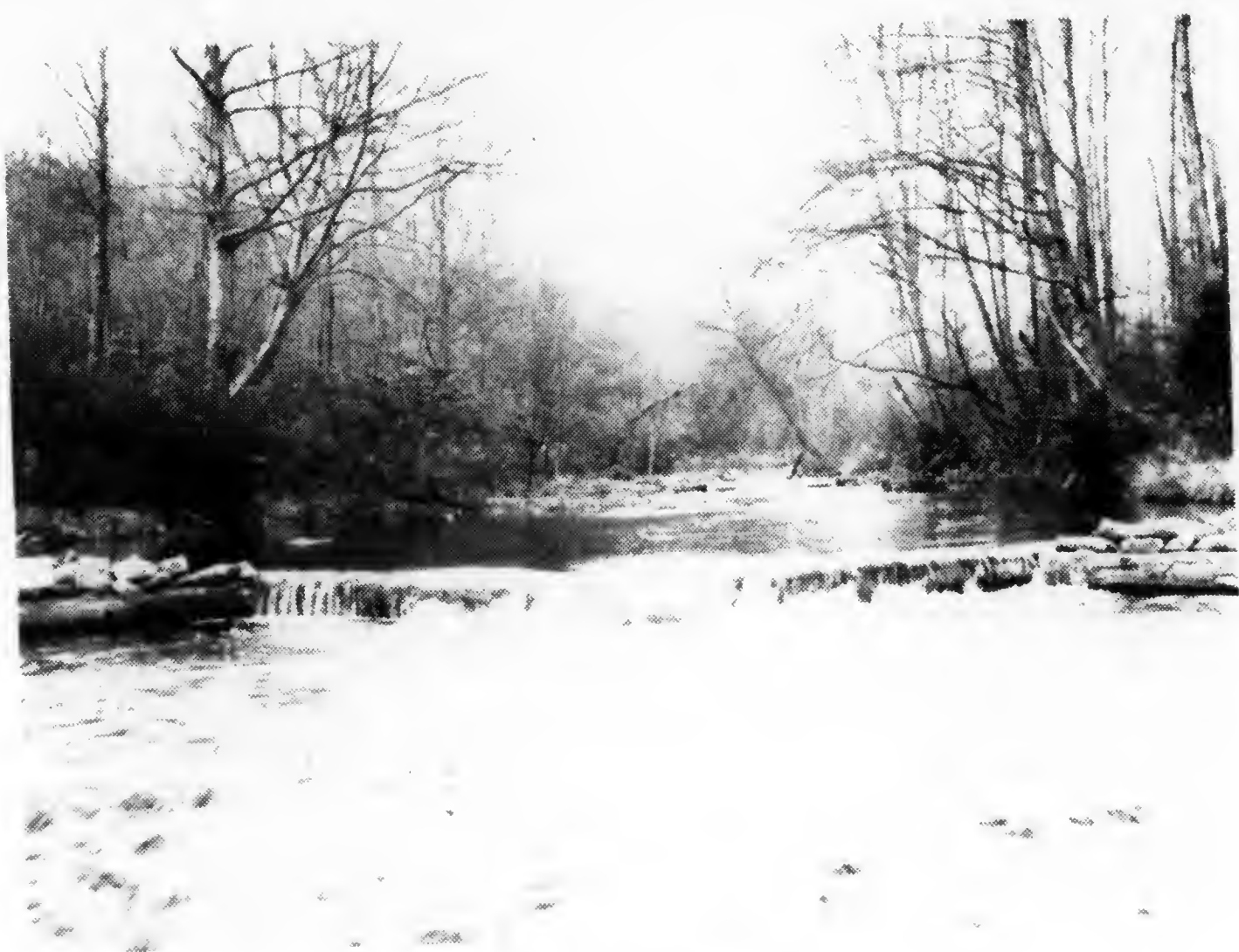
BEAR CREEK DAM No. 33
