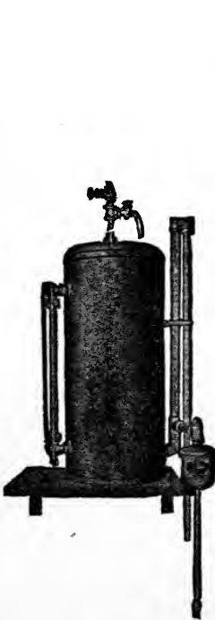
Automatic Gas Sampler and Combined \text{CO}_2 and Draft Recorder designed by the Author
