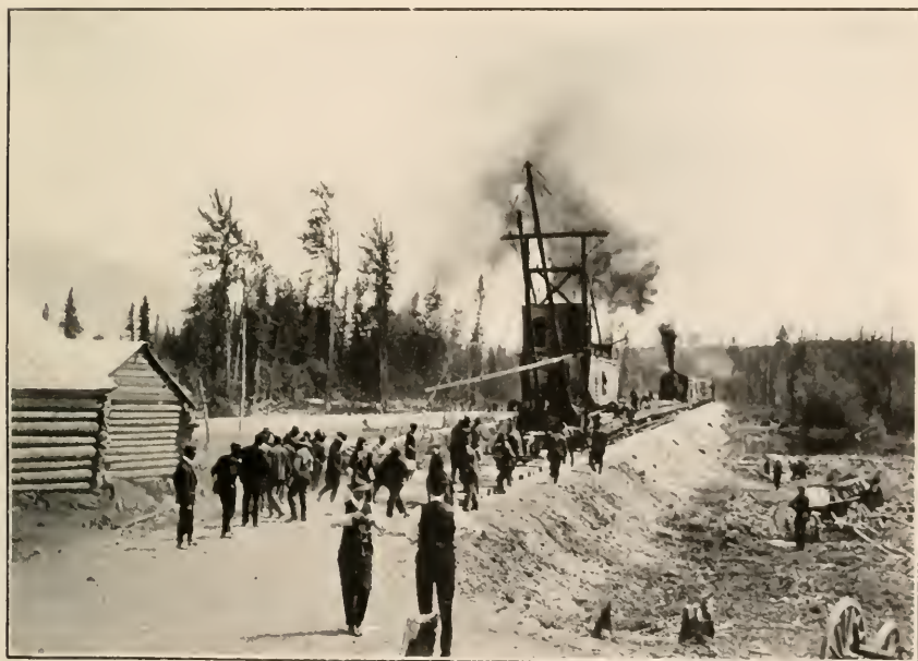
LAYING RAILS, TÊTE JAUNE, B. C., JULY 17, 1912
