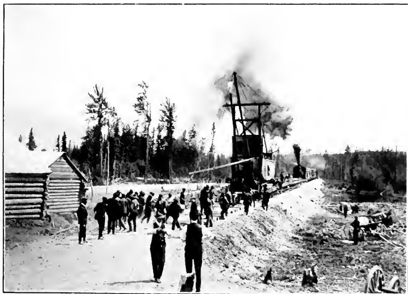
LAYING RAILS, TÊTE JAUNE, B. C., JULY 17, 1912
