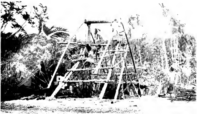
Rebuilding the village after a hurricane
