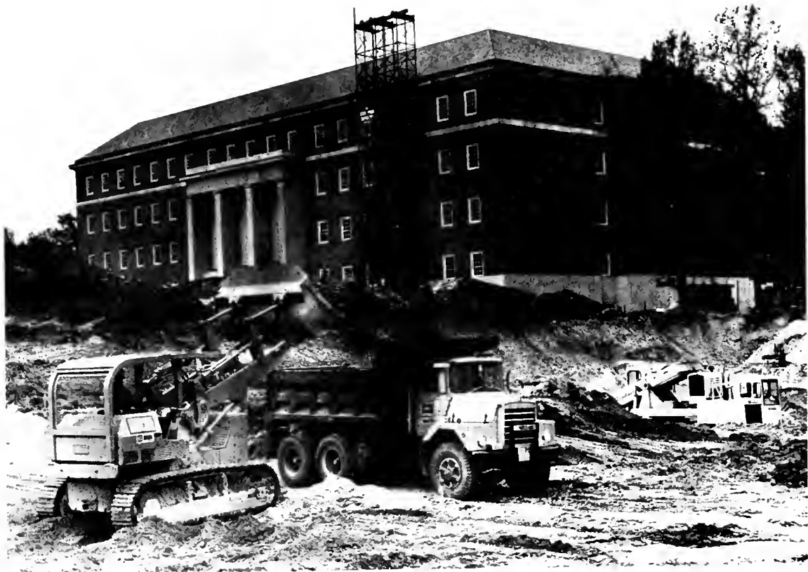
The new Zoology-Psychology Building receives the finishing touches of construction as ground is broken, in the foreground, for the new undergraduate library at College Park.
