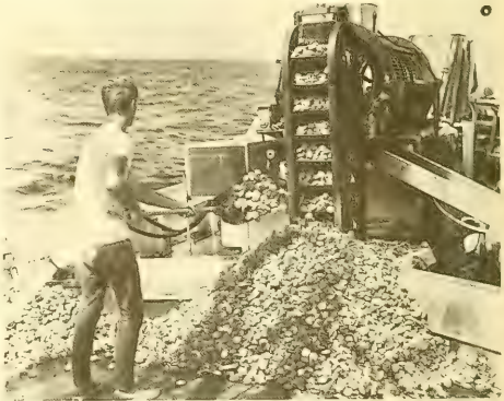
Fig. 5 - Feeding the bucket conveyor leading to "separator."
