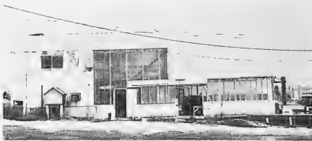
Fig. 3 - Oyster hatchery at Bayville, Oyster Bay, Long Island, N.Y., is capable of producing 3,000 to 6,000 bushels of seed oysters a year. This hatchery began to rear spat as singles in 1969. Transparent roof and walls allow sunlight to reach tank cultures of algae.
