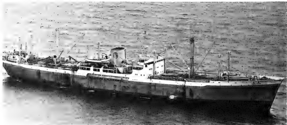
Fig. 7 - The South Korean factory ship 'Shin Hung'. Built in Norway in 1947, she was operated by the Norwegians as the refrigerated processor 'Bataan' until 1967, then sold to Shin Hung Refrigeration Co. The Shin Hung is 508 feet long, 7,073 gross tons, with a crew of 200. She first appeared off Alaska in 1969, processing salmon and bottom fish catches from 7 trawlers and 5 gillnetters. She is equipped with: 1) a complete two-line canning plant (10 ton an hour capacity); 2) a reduction plant (25 ton daily capacity); 3) a sharp freezer (100 ton daily capacity); 4) refrigerated holds with a 2,900 ton capacity; and storage space for 400 tons of fish meal, 200 tons of fish oil, and 2,500 tons of canned fish.
