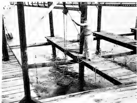
Fig. 2 - Photograph of monorails, movable block and tackle, and chicken wire cover arrangement of bridle on tray.
