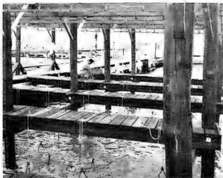
Fig. 1 - Overall view of tray rack showing construction of walks and position of superstructure.
