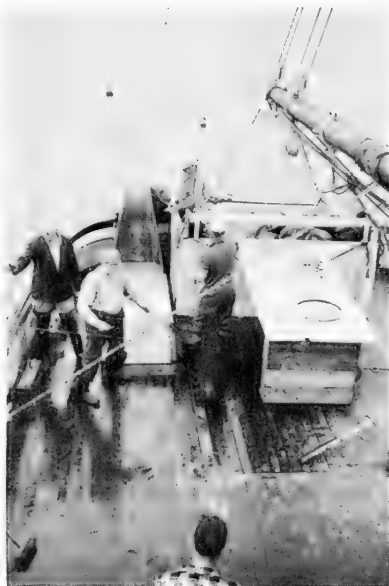
FIG. 9 - SNAPPING THE GANGIONS ON THE STAINLESS STEEL LONG LINE AS IT PAYS OUT OVER THE CHUTE AT STERN. TABLE AT RIGHT WAS USED FOR BAITING.
